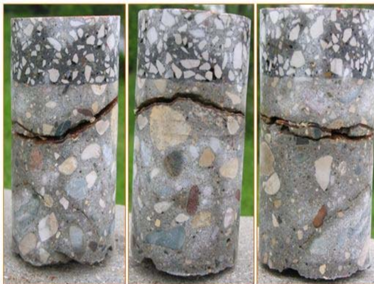
Figure 65. Three views of Core #2, which appeared as “epoxy-filled delamination” in field (raw) GPR data.
