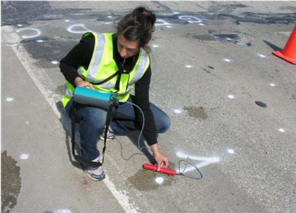
Figure 98. ER measurement on EB lane along Line C (5ft from curb), 10ft from west abutment, near origin.
