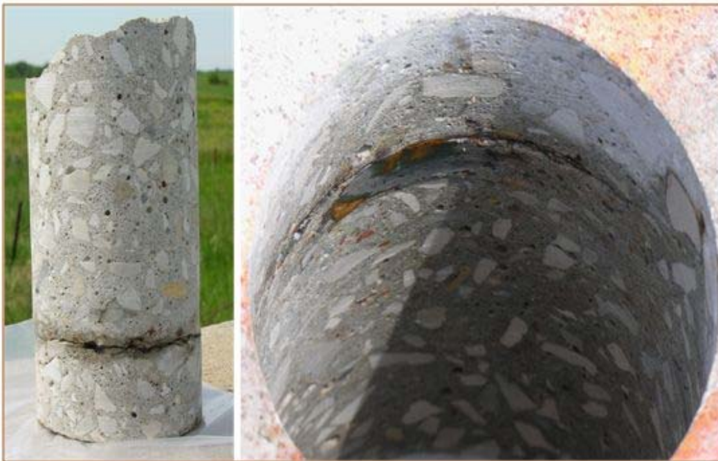
Figure 100. Core #1 – expected to be “fair to poor” – shows delamination, and core hole reveals “nicked” rebar, delamination and corrosion.
