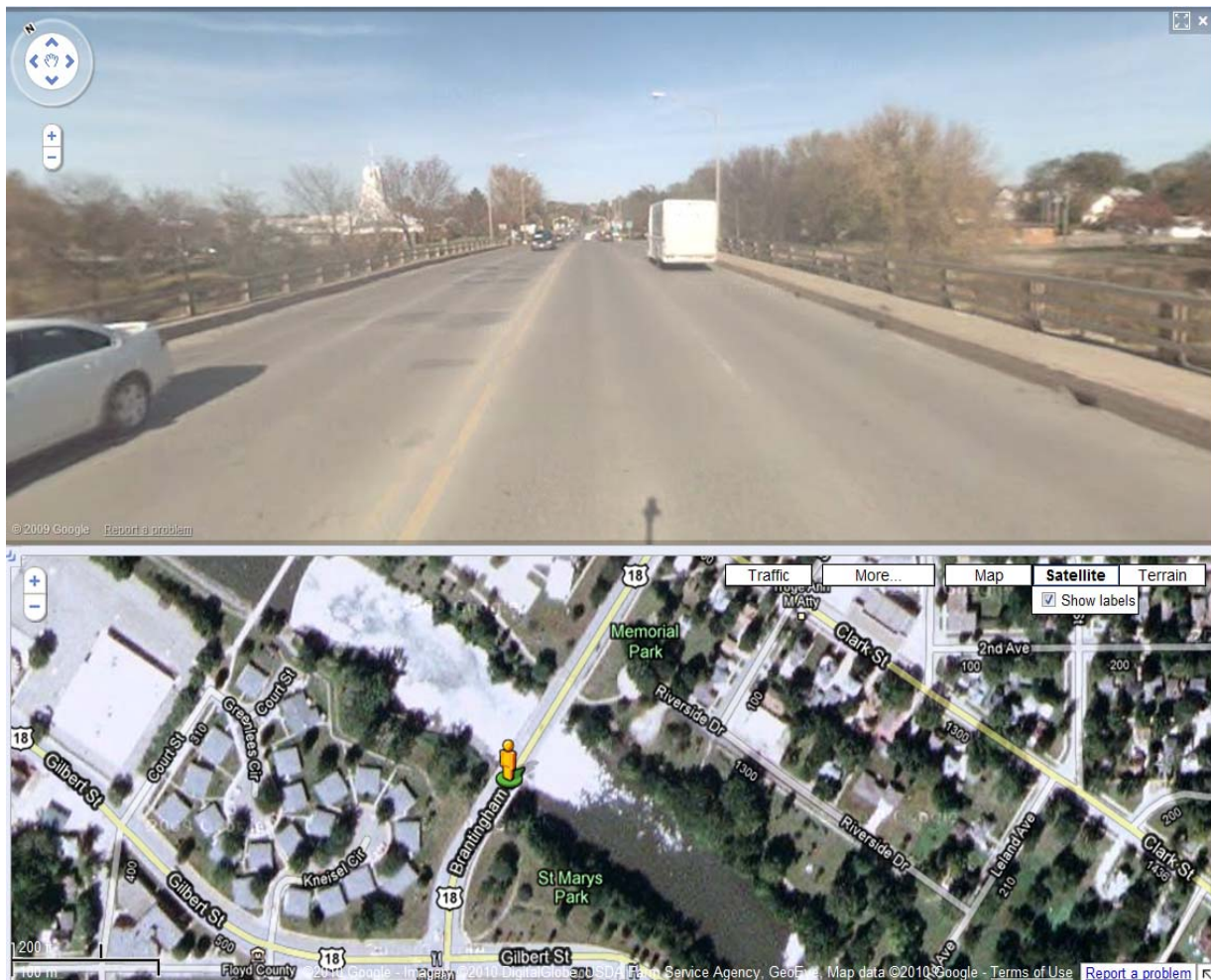
Figure 83. Google map street view in EB direction, on Deck O4 crossing the Cedar River.
