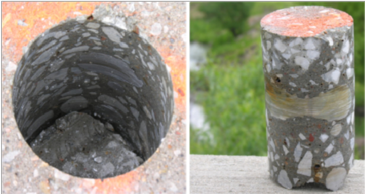
Figure 110. Core #1 – rated “good” – reveals no damage; core hole shows part of sliced upper rebar along with imprint of lower rebar.
