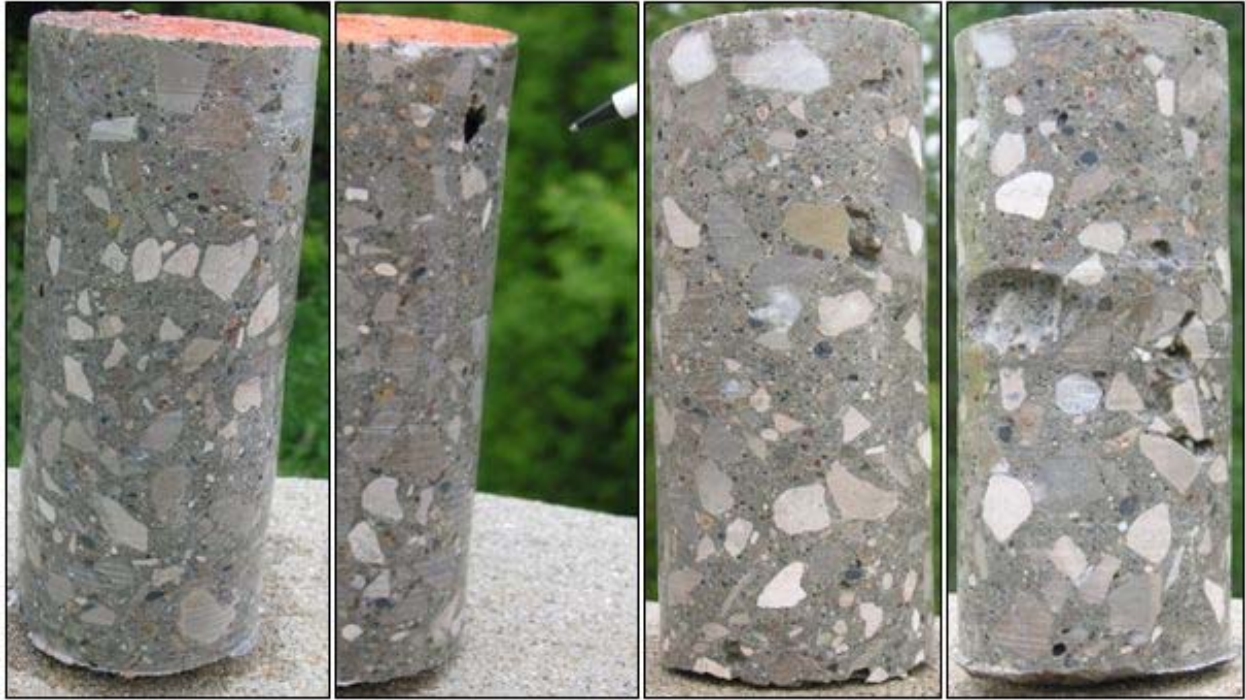
Figure 82. Cores 1 through 4 (left to right), where Core 1 is “control” and Cores 2 to 4 selected where GPR signal looked “slightly worse”, yet not obviously deteriorated. Note pen-sized vug in Core #2.
