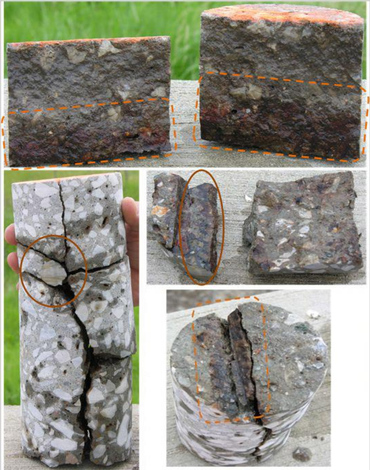
Figure 112. Core #3, retrieved in six pieces, extracted above longitudinal bar at surface crack.
