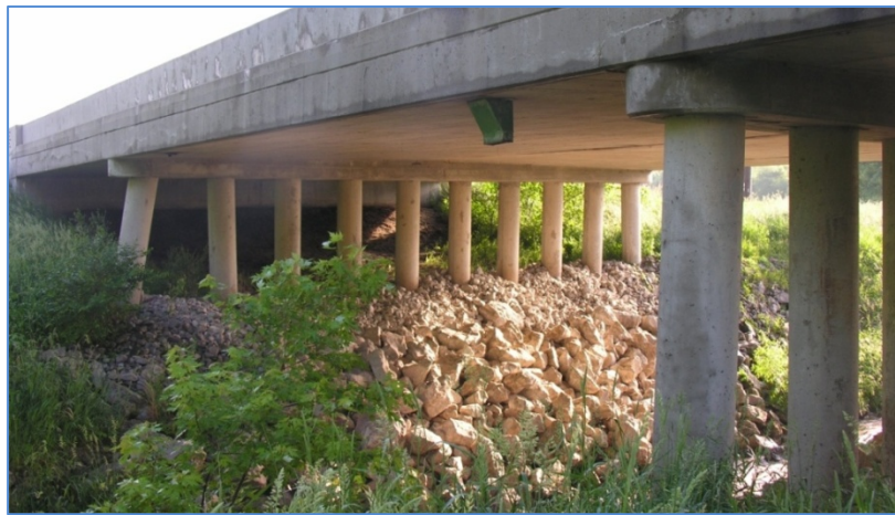
Figure 75 Side view of Bridge O3 showing full-depth (slab) deck construction between piers
