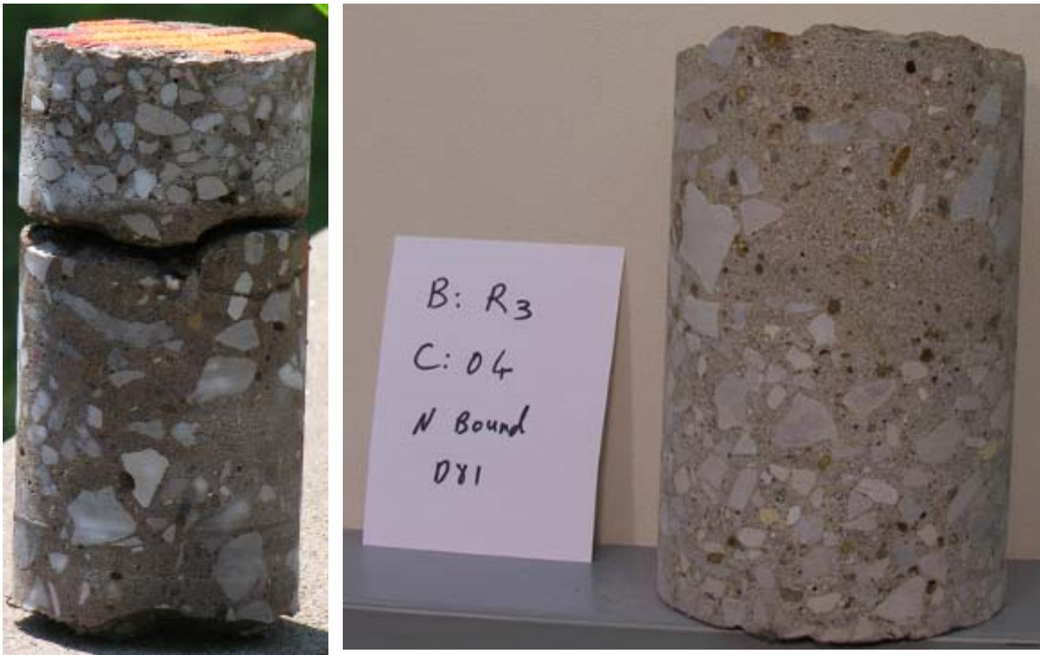
Figure 140. Cores 3 (left) and 4 (right), graded “serious” and “fair to poor” with IE.
