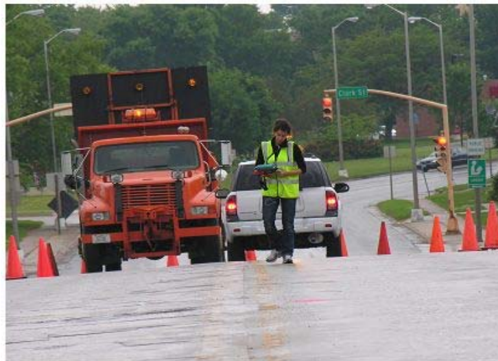
Figure 85. Simultaneous electrical resistivity measurements being taken on east end of deck.
