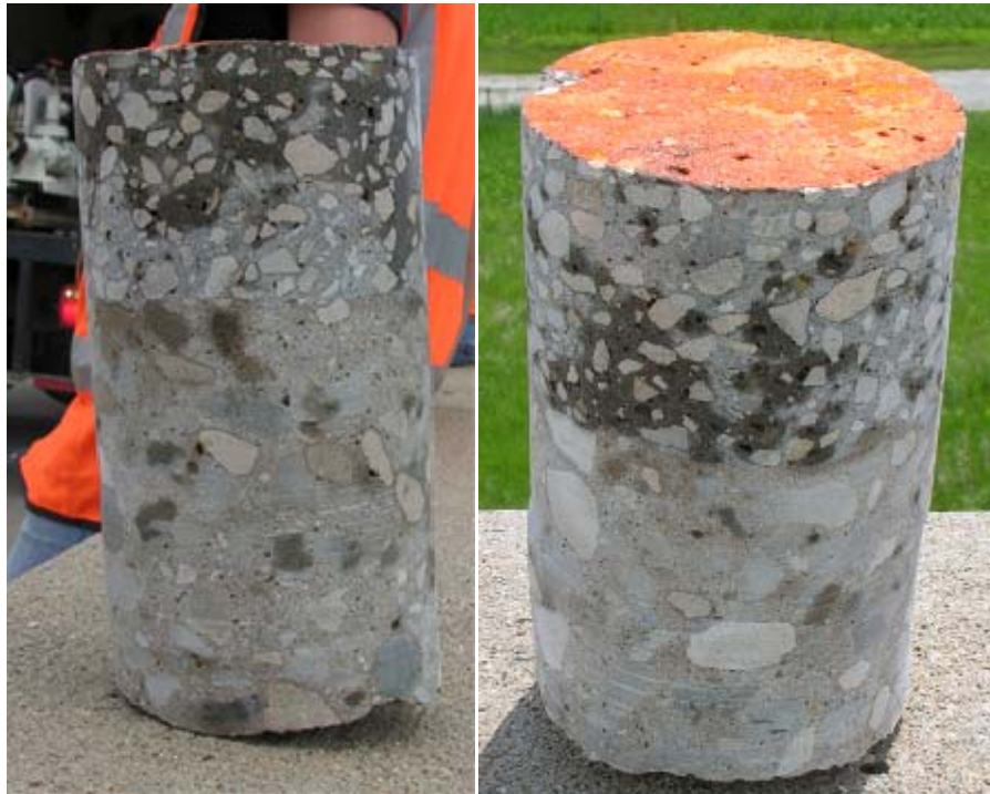
Figure 132. Cores 3 (left) and 4 (right), graded “deteriorated” and “good” with GPR.
