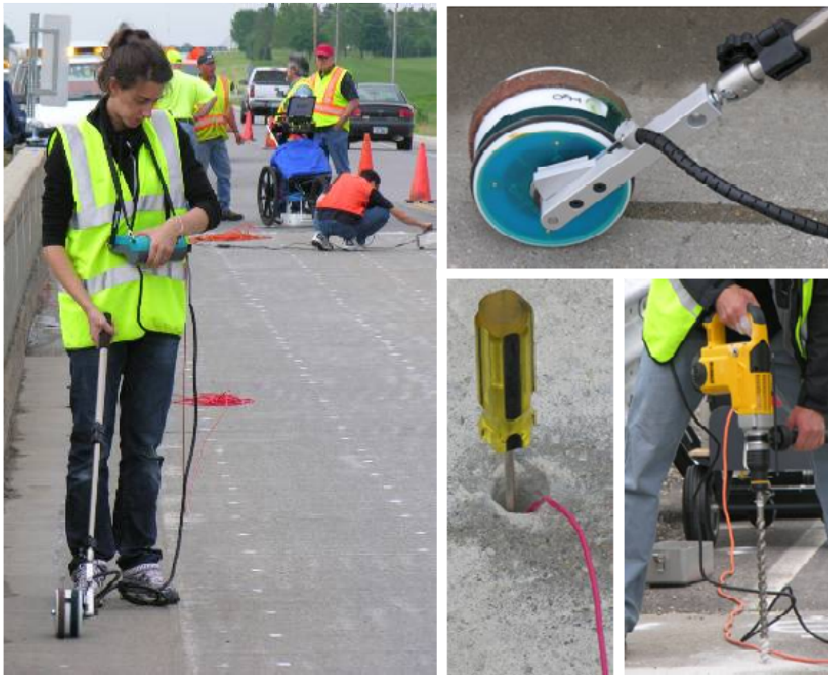
Figure 51. Half-cell (HC) potential measurement on deck; showing probe detail, drilled hole and wire lead connected electrically to the upper rebar mat.
