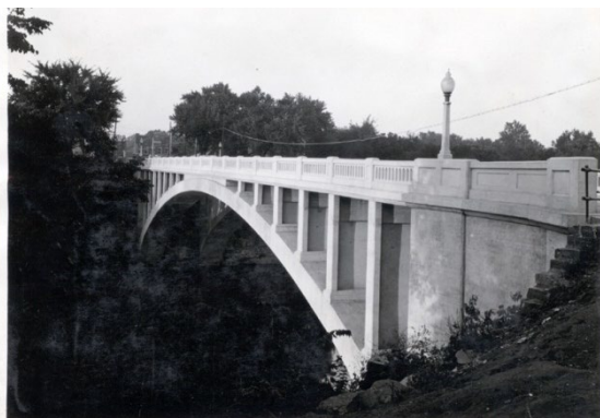
Figure 2.3.2-1 Original Concrete Arch Bridge
