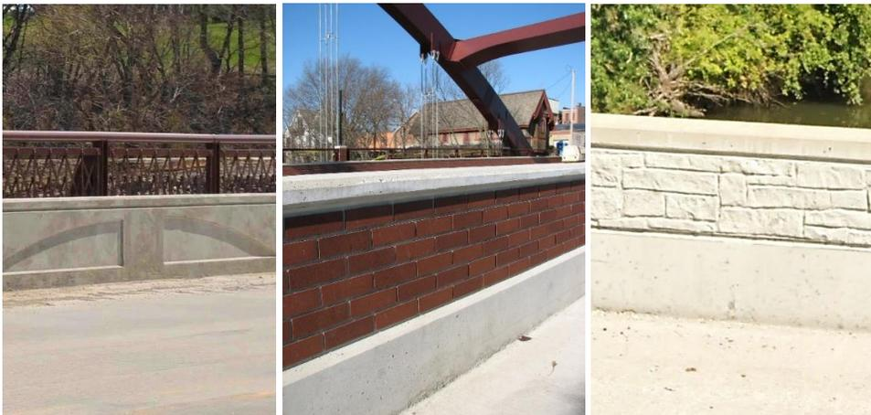
**Figure 5.8.1.2.5-4. Examples of Barrier Traffic Face Treatments**
