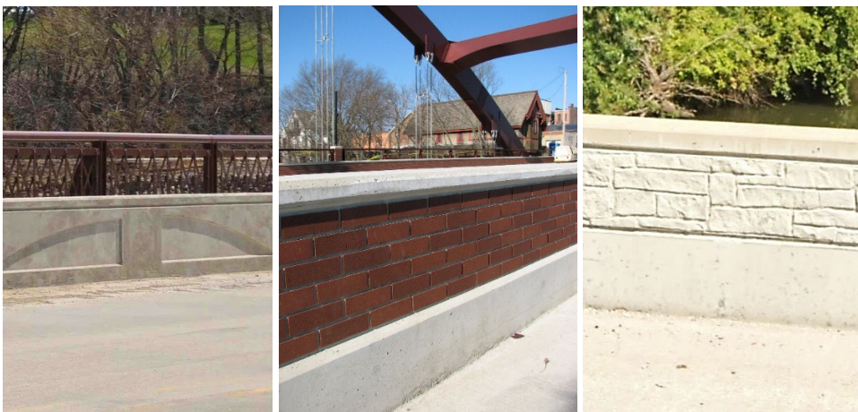
Figure 5.8.1.2.5-4. Examples of Barrier Traffic Face Treatments
