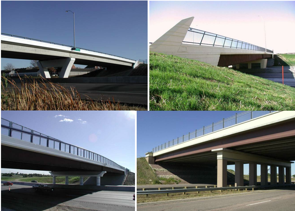
Figure 9.4.3. Level “B” bridge examples in Iowa
