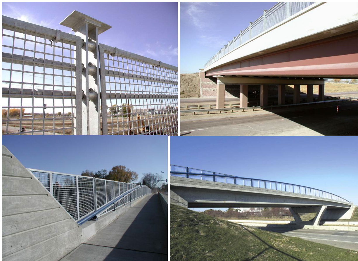
Figure 9.5.3.7-2. Bridges with complementary bolt-on aesthetic details
