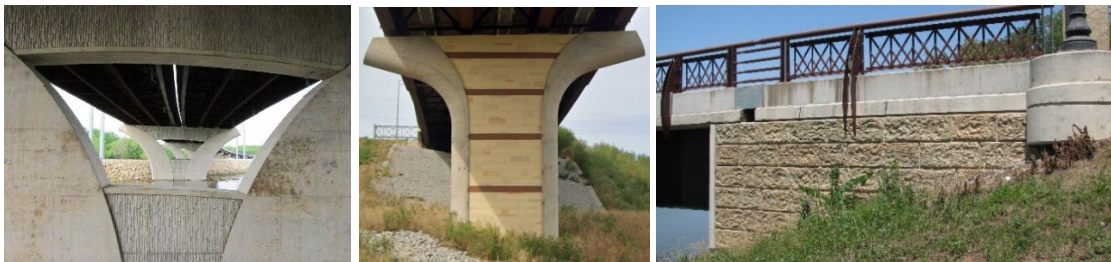
Figure 9.5.9.4. Examples of form liner concrete texture
