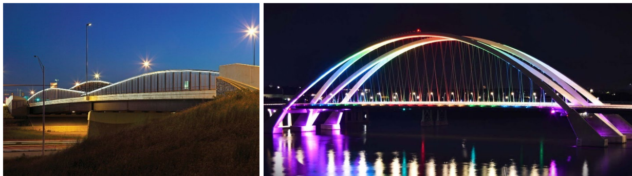
Figure 9.5.8. Examples of City-installed lighting
