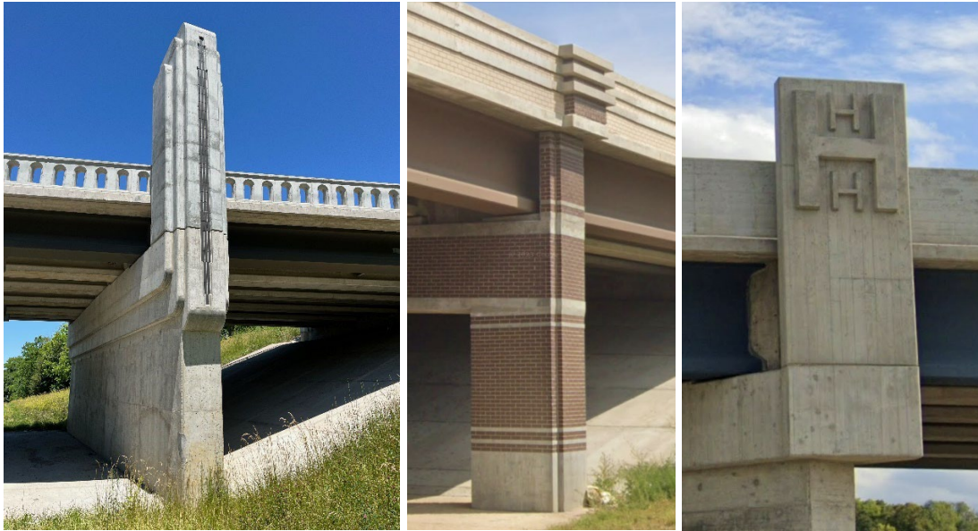
Figure 9.5.5.2-2. Examples of pier cap-supported aesthetic elements
