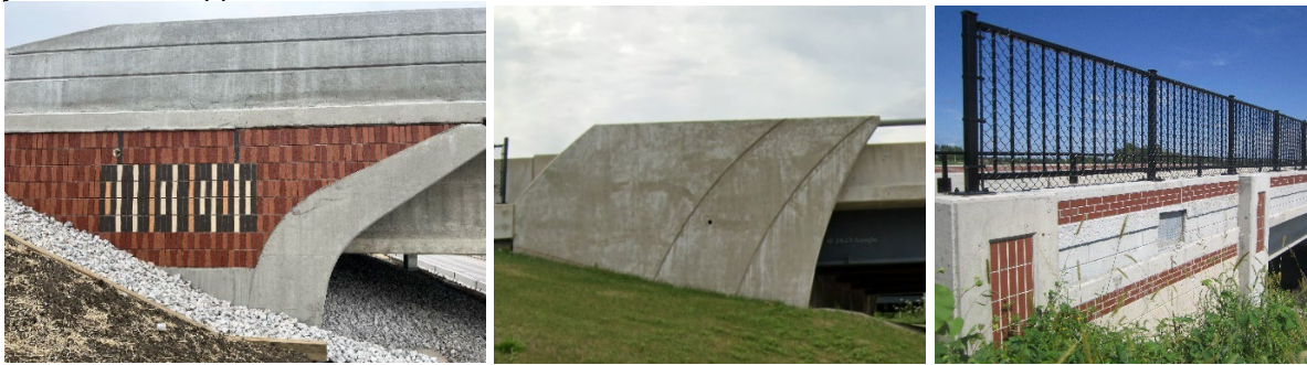
Figure 9.5.5.4-1. Examples of abutment wingwalls with no exposed vertical construction joints
