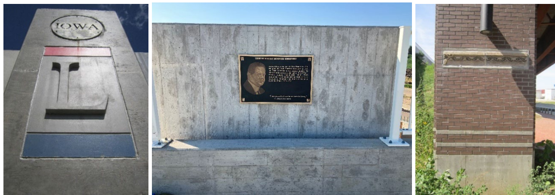
Figure 9.5.9.8.3. Examples of decorative prefabricated inserts
