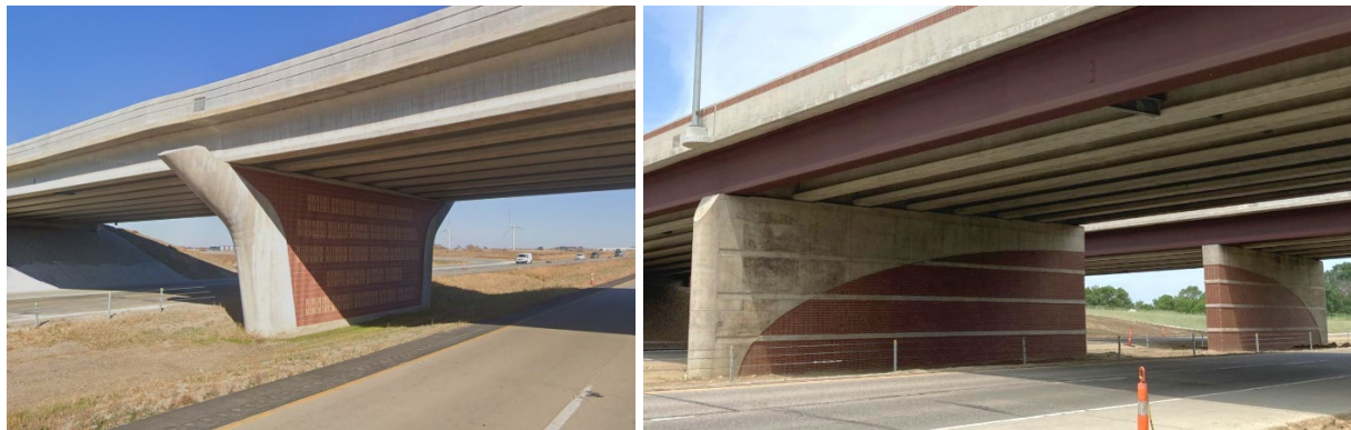
Figure 9.5.5.2-1. Examples of enhanced pier shapes that meet collision force requirements
