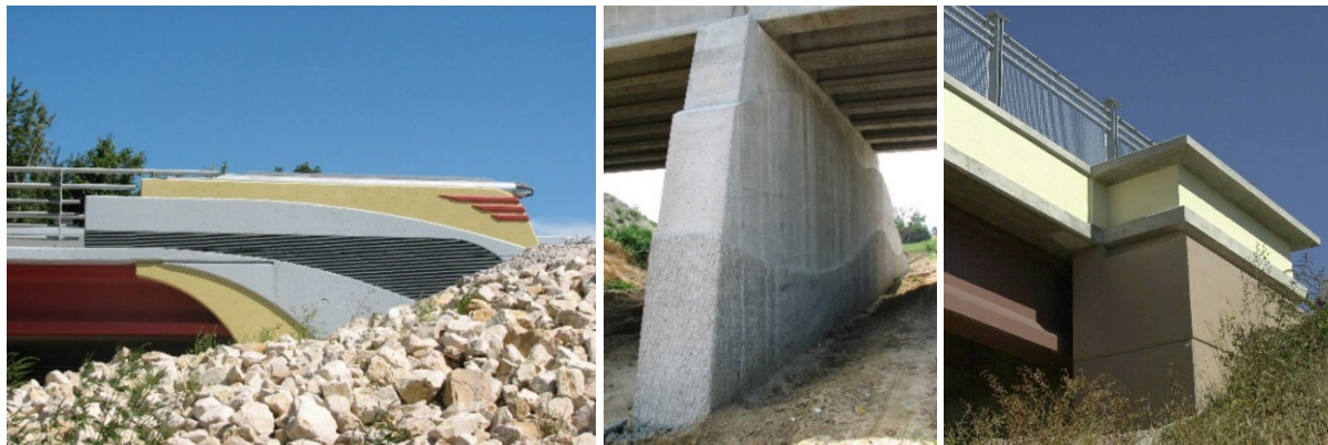
Figure 9.5.9.2. Examples of concrete surface articulation
