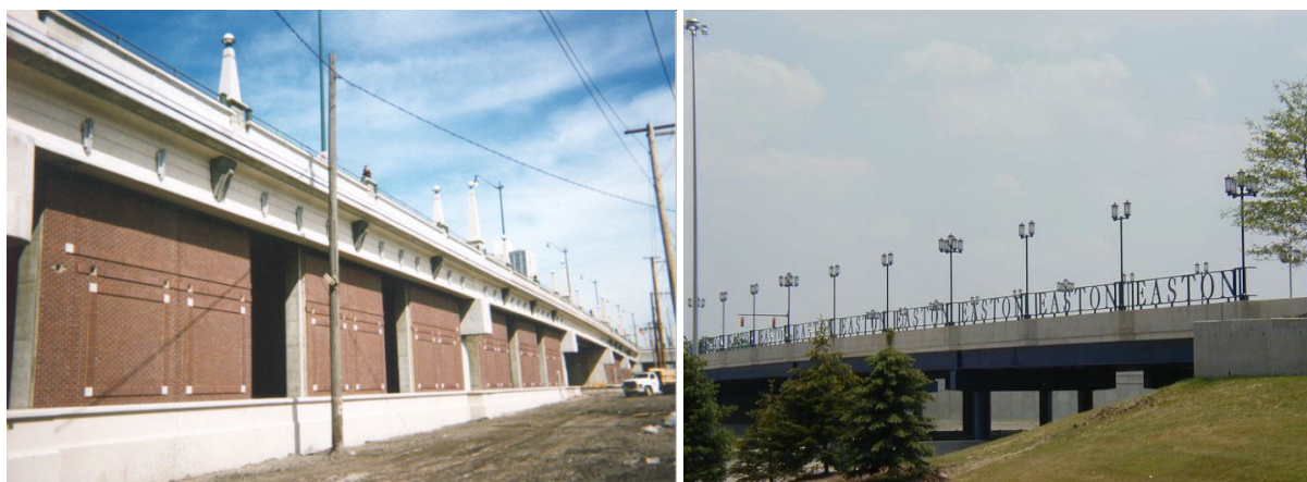
Figure 9.5.3.7-1. Bridges with ineffective bolt-on aesthetic details
