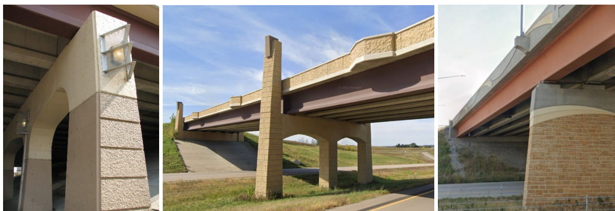
Figure 9.5.10.2. Examples of painted bridge surfaces
