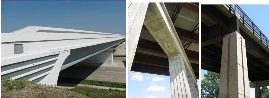
Figure 9.5.9.3. Examples of concrete surface rustication
