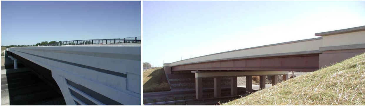
Figure 9.5.3.1. Bridges with long, slender appearance
