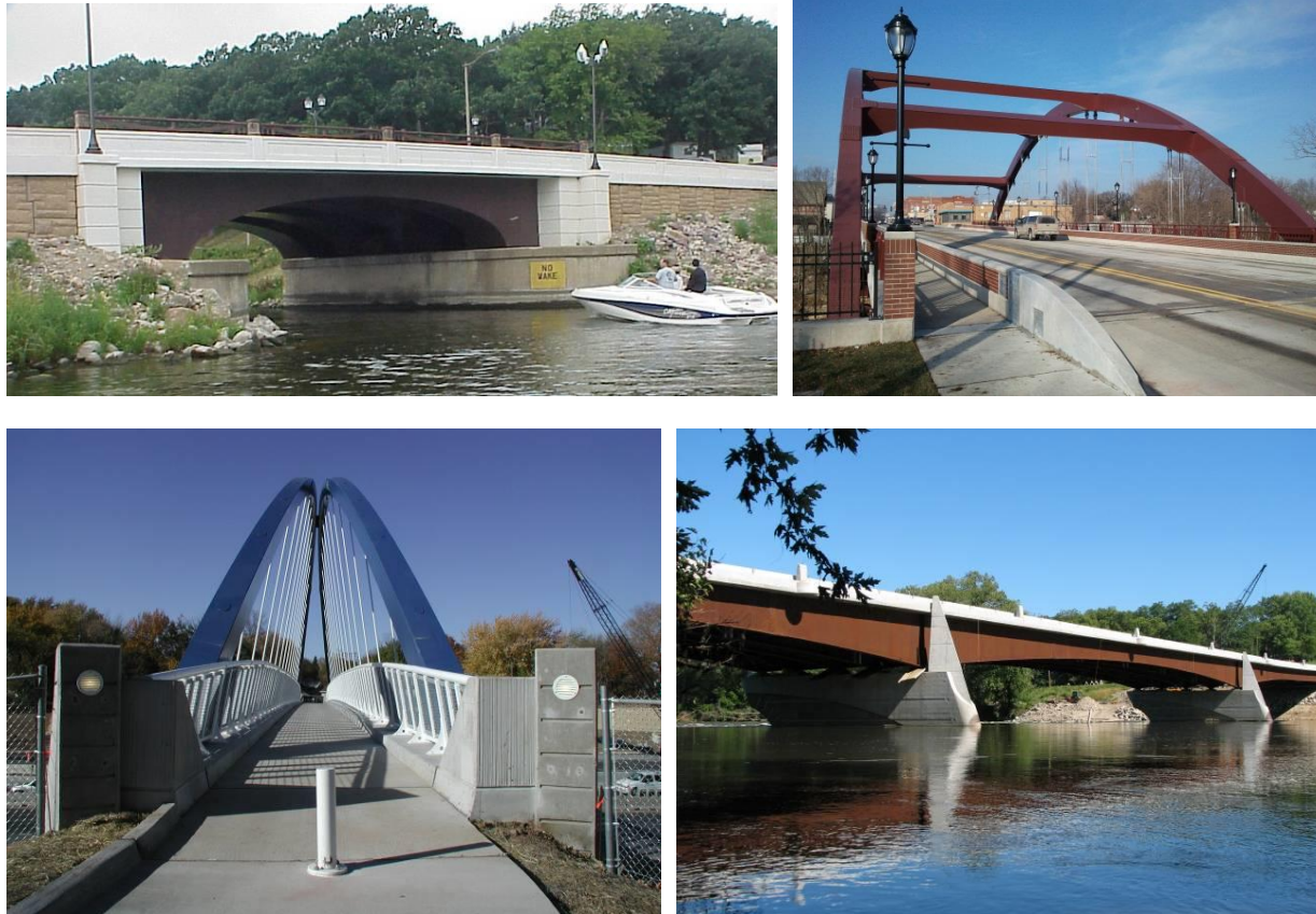
Figure 9.4.4. Level “A” bridge examples in Iowa
