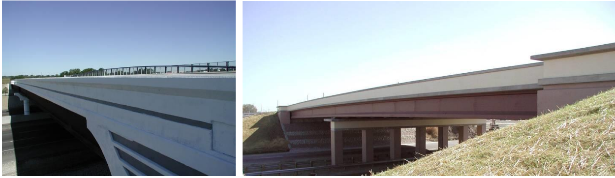
Figure 9.5.3.1. Bridges with long, slender appearance
