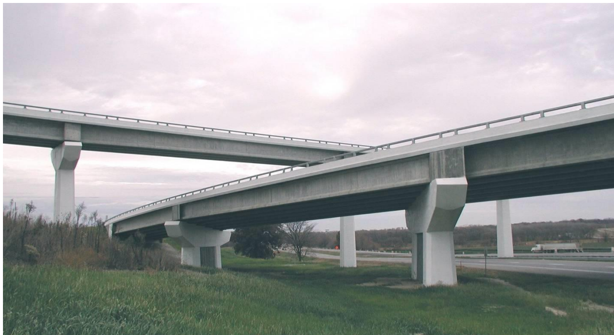
Figure 9.5.3.4. Bridges with minimal column count
