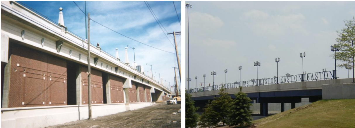
Figure 9.5.3.7-1. Bridges with ineffective bolt-on aesthetic details
