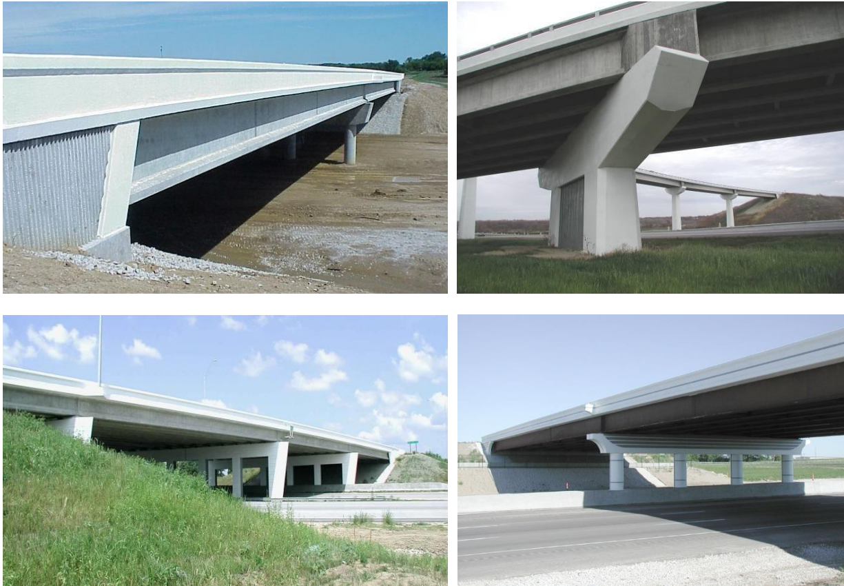
Figure 9.4.2. Level “C” bridge examples in Iowa
