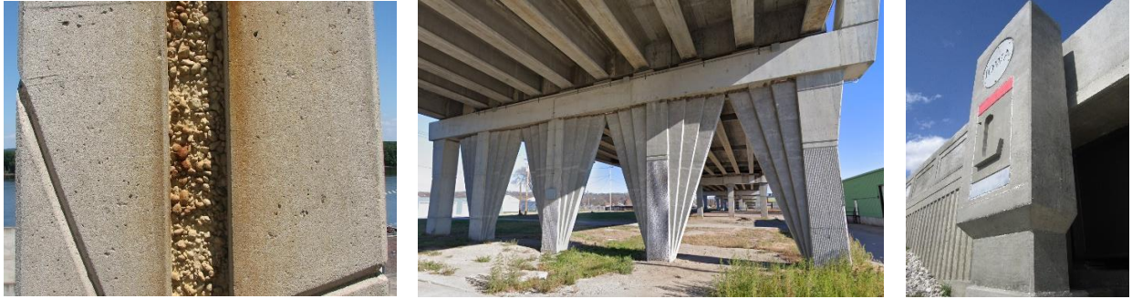
Figure 9.5.9.8.1. Examples of abrasive blast finished concrete surfaces
