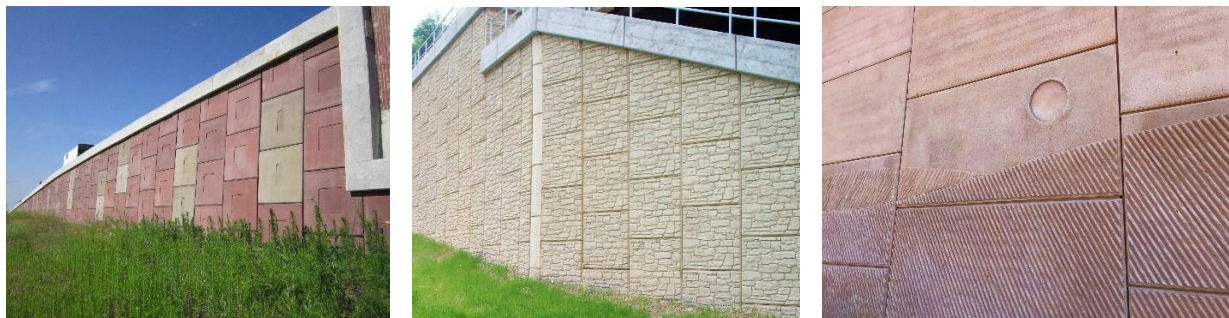
Figure 9.5.9.6. Examples of integrally colored MSE wall panels
