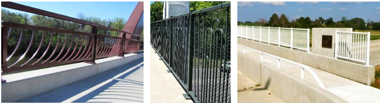
Figure 9.5.11.2. Examples of powder coated galvanized (duplex system coated) steel railings
