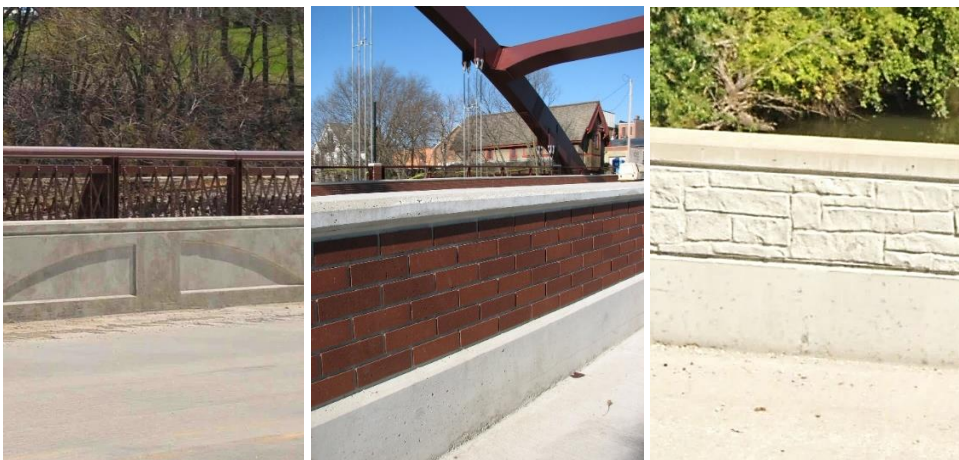
Figure 5.8.1.2.5-4. Examples of Barrier Traffic Face Treatments
