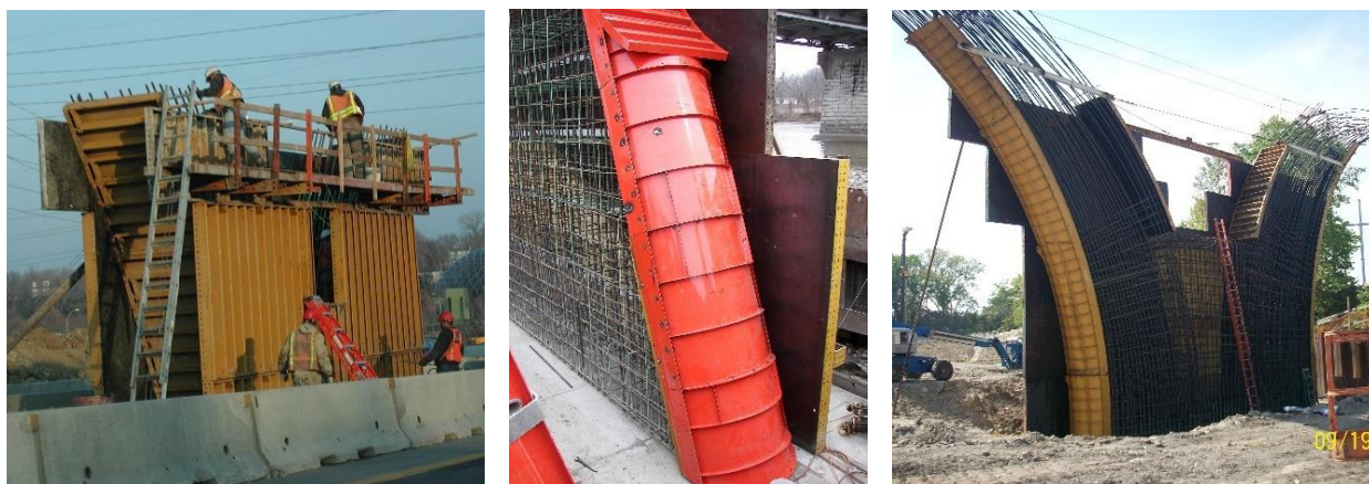
Figure 9.5.5.3-1. Examples of formwork used to create special pier shapes
