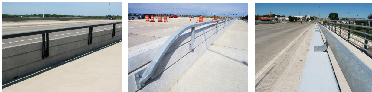
Figure 9.5.11.1-2. Examples of painted and unpainted galvanized bicycle railing attachments
