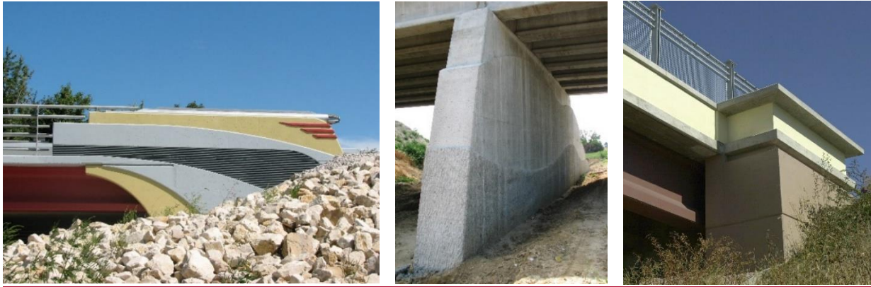
Figure 9.5.9.2. Examples of concrete surface articulation
