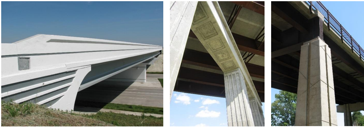
Figure 9.5.9.3. Examples of concrete surface rustication
