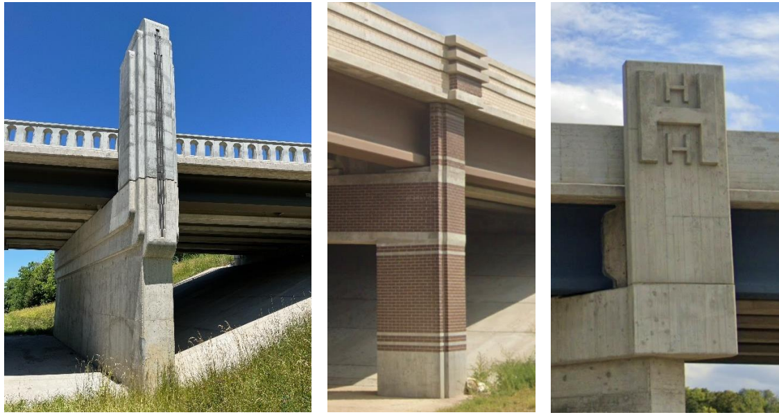
Figure 9.5.5.2-2. Examples of pier cap-supported aesthetic elements
