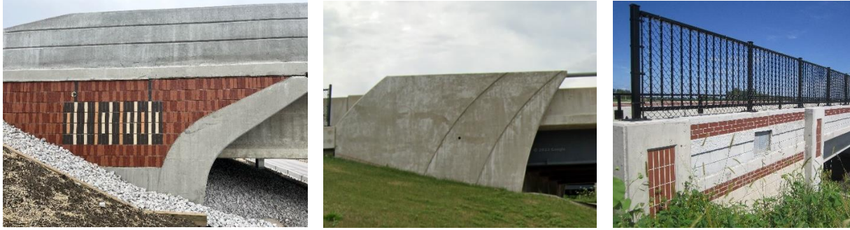
Figure 9.5.5.4-1. Examples of abutment wingwalls with no exposed vertical construction joints
