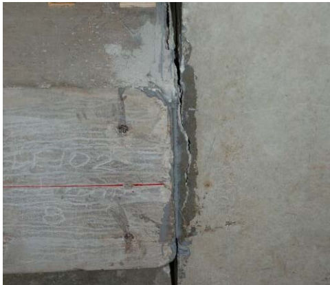
(a) Side view of the failed specimen
