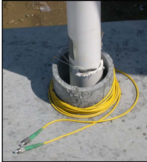
Figure 4. Fiber optic sensors left in position on completed bridge
