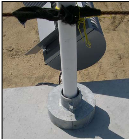
Figure 5. Galvanized trumpet pipe cover provides UV protection for FBG sensors leads
