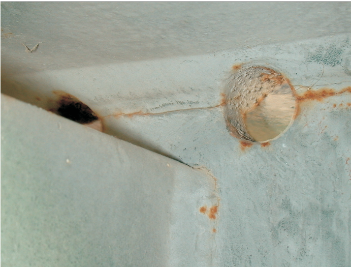
Photo 1: Drilling to Arrest Fatigue Cracks
