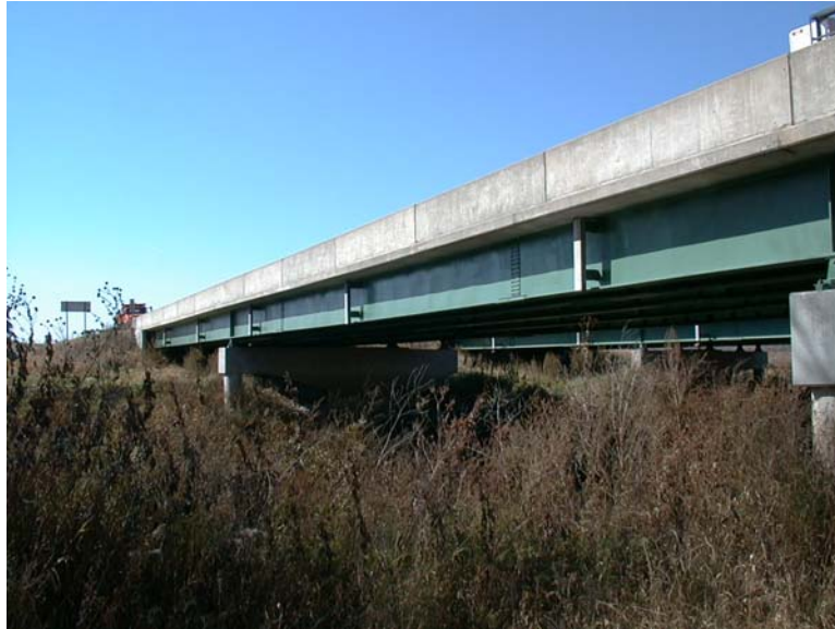
a. Bridge 5075.5R080 looking northwest.
