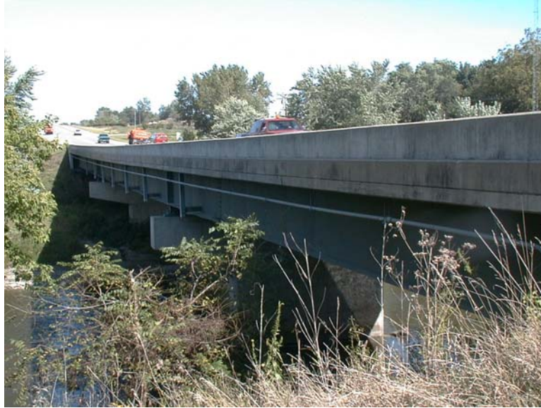
a. Bridge 4048.2S017 looking northeast
