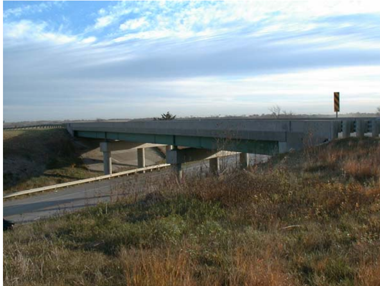
a. Bridge 2700.0R035 looking northeast.
