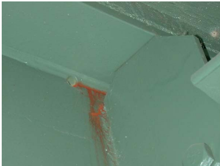
b. Typical drilled hole retrofit in a web.
