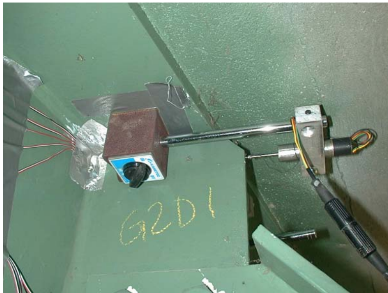
b. Typical out-of-plane displacement instrumentation (bridge 5075.5R080 shown).
