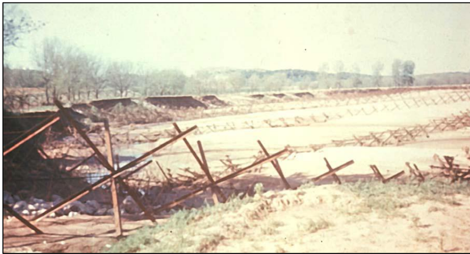
Figure 10. Kellner jacks used to redirect flow patterns (Bradley et al. 2005)
