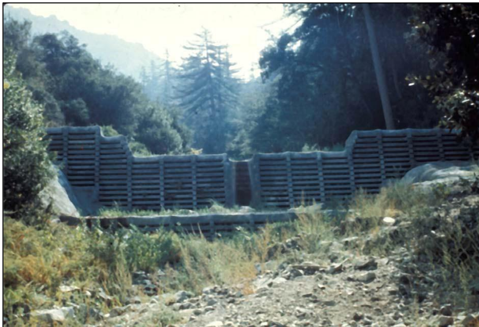
Figure 7. Debris basin constructed of precast concrete sections (Bradley et al. 2005)
