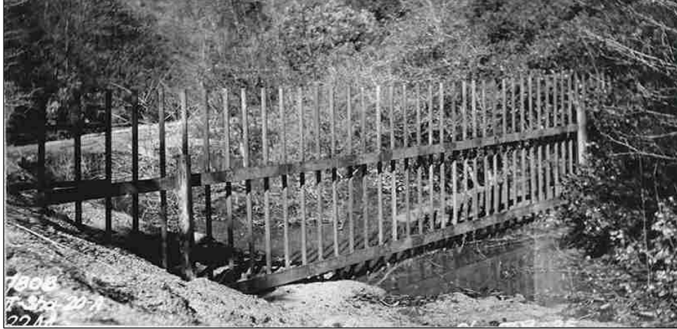
Figure 19. Debris rack installed upstream (Bradley et al. 2005)
