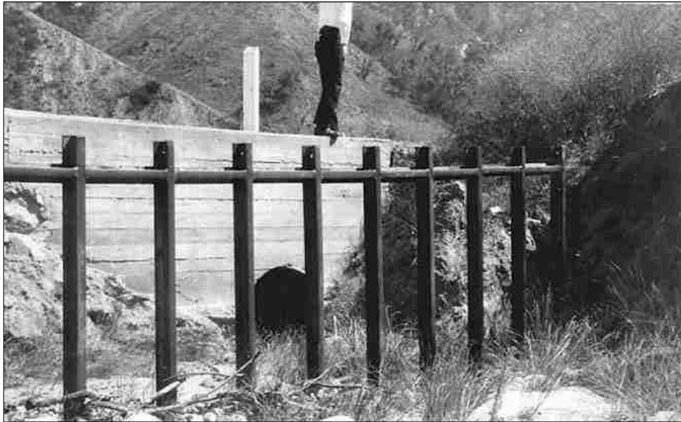
Figure 20. Steel debris rack (Bradley et al. 2005)
