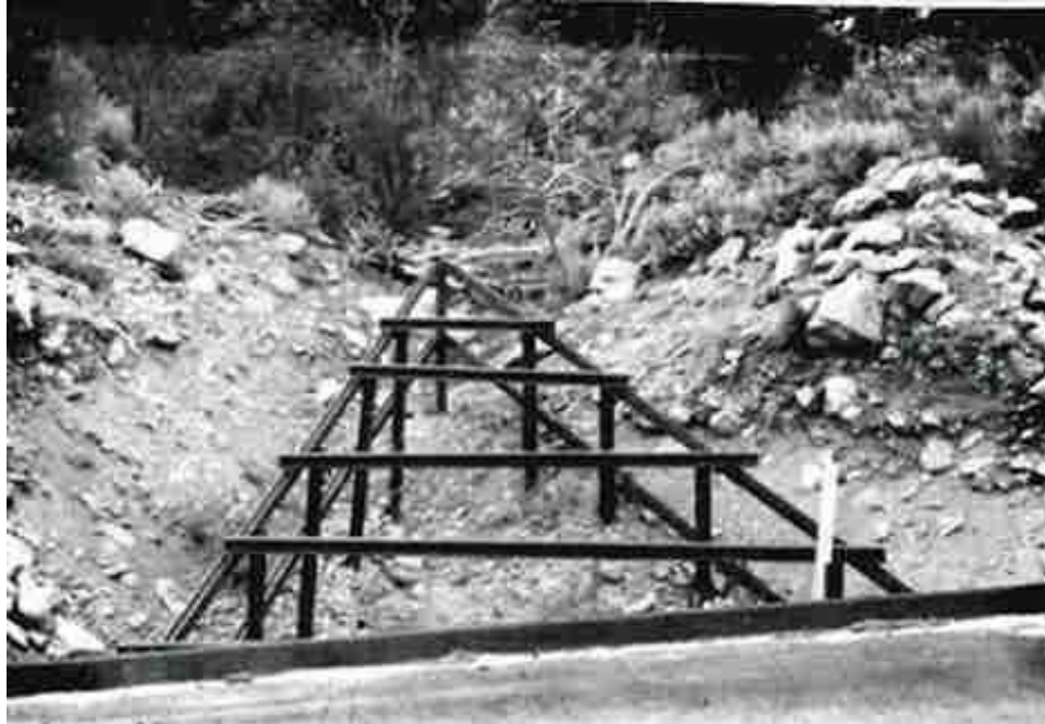
Figure 11. Debris deflector looking upstream (Bradley et al. 2005)
