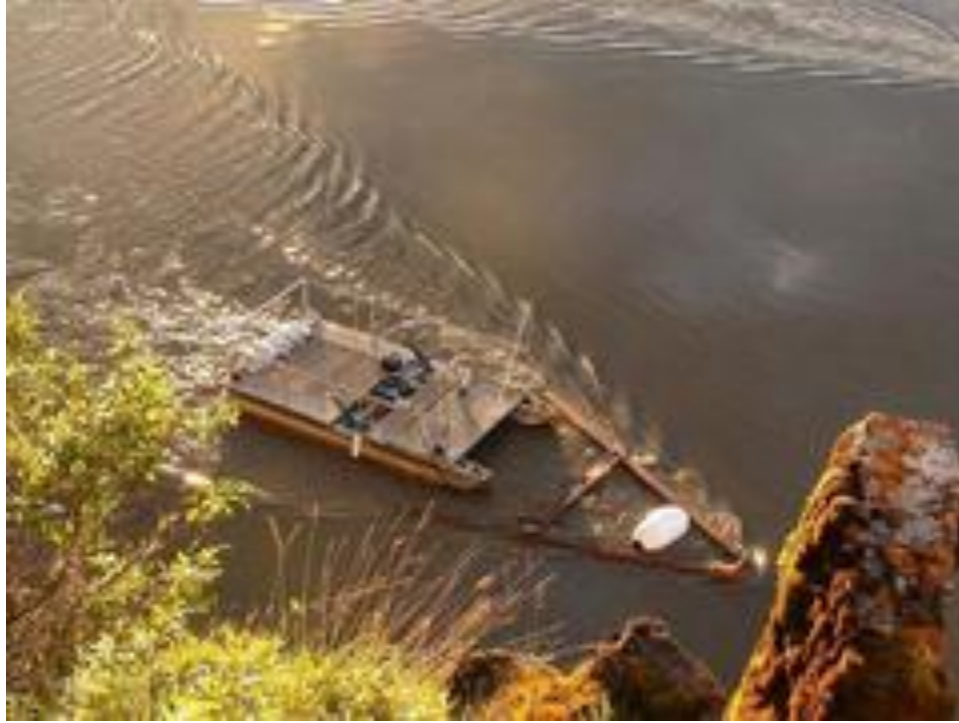
Figure 18. Debris boom protecting surface turbine (Tyler 2011)
