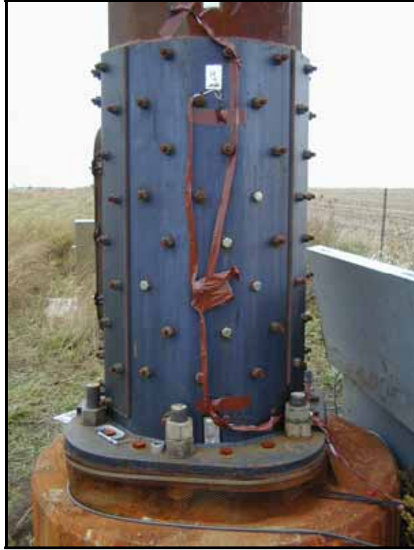
Figure 1.1 – Jacket retrofit designed by Wiss, Janney, Elstner, and Associates and installed in Clear Lake, Iowa
