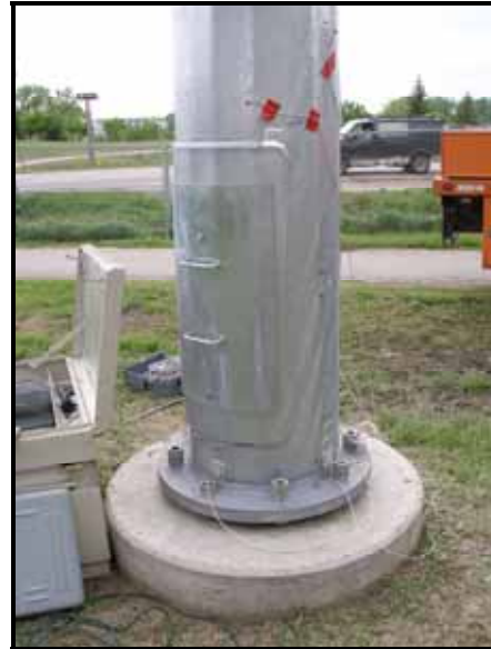
(b) Retrofit tower
