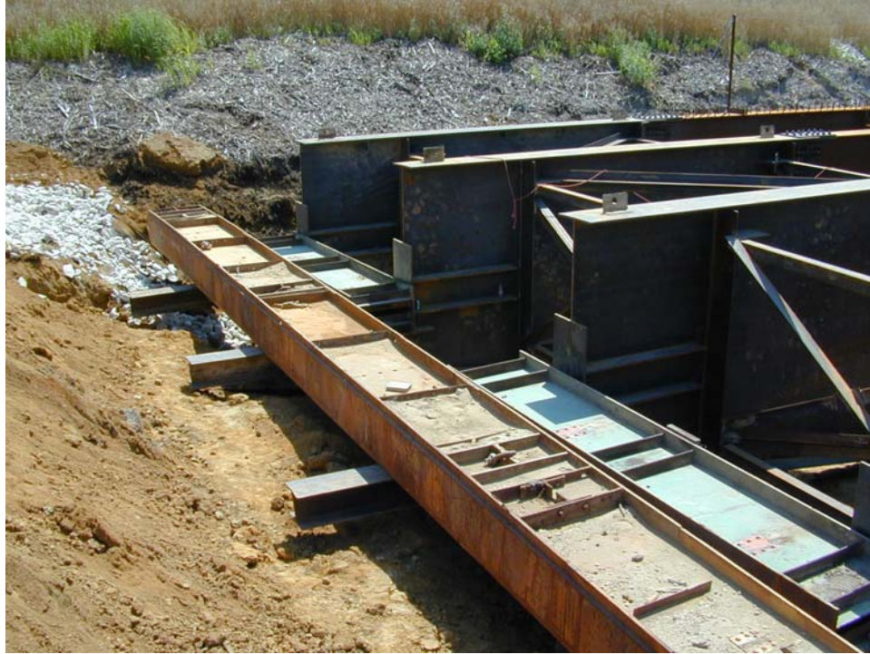
Figure 3.12. Spreader beams located between the tugger beam and the tail section.
