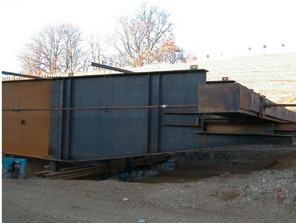
Figure 3.6. Tapered launching tail attached to the girder system.
