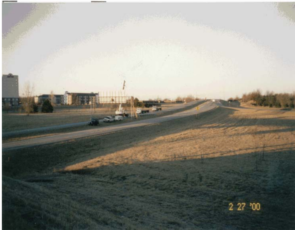
a. Overview of the Sign Truss Site
