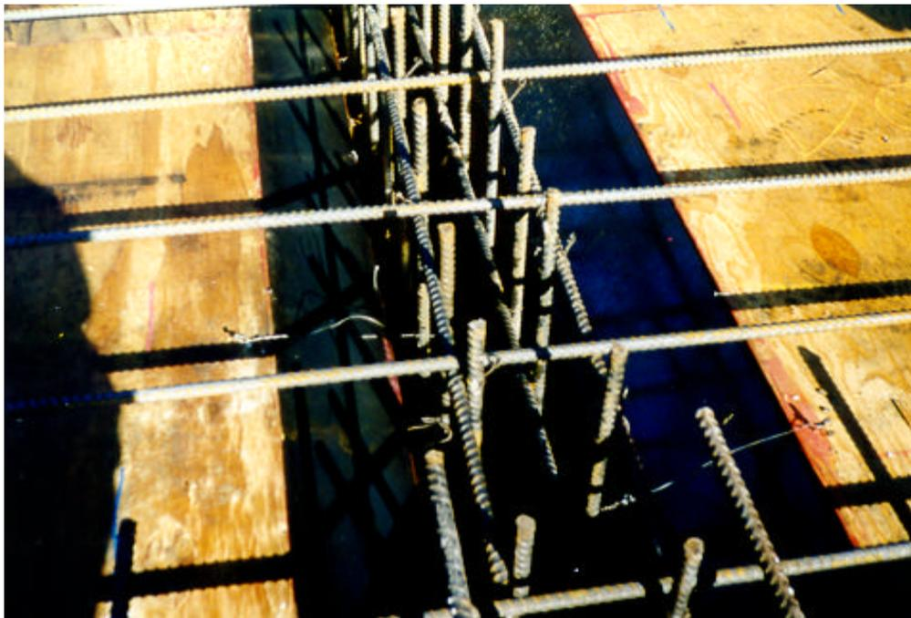
The vertical wall steel is properly secured to prevent it from drifting inward.
