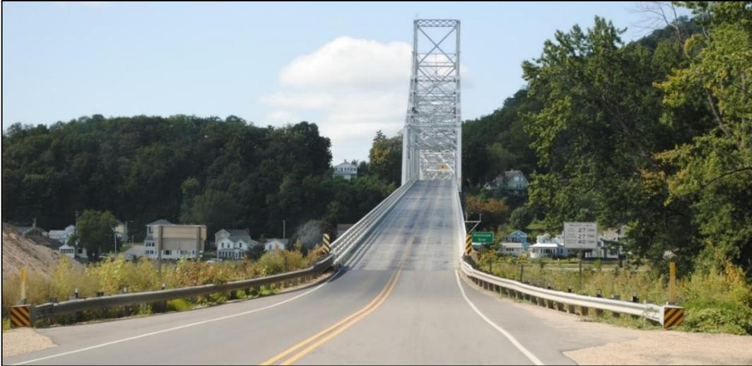
**Figure 13. View of approach span deck and east through truss from causeway, looking west. Residences of Lansing, Iowa are visible beyond.**
