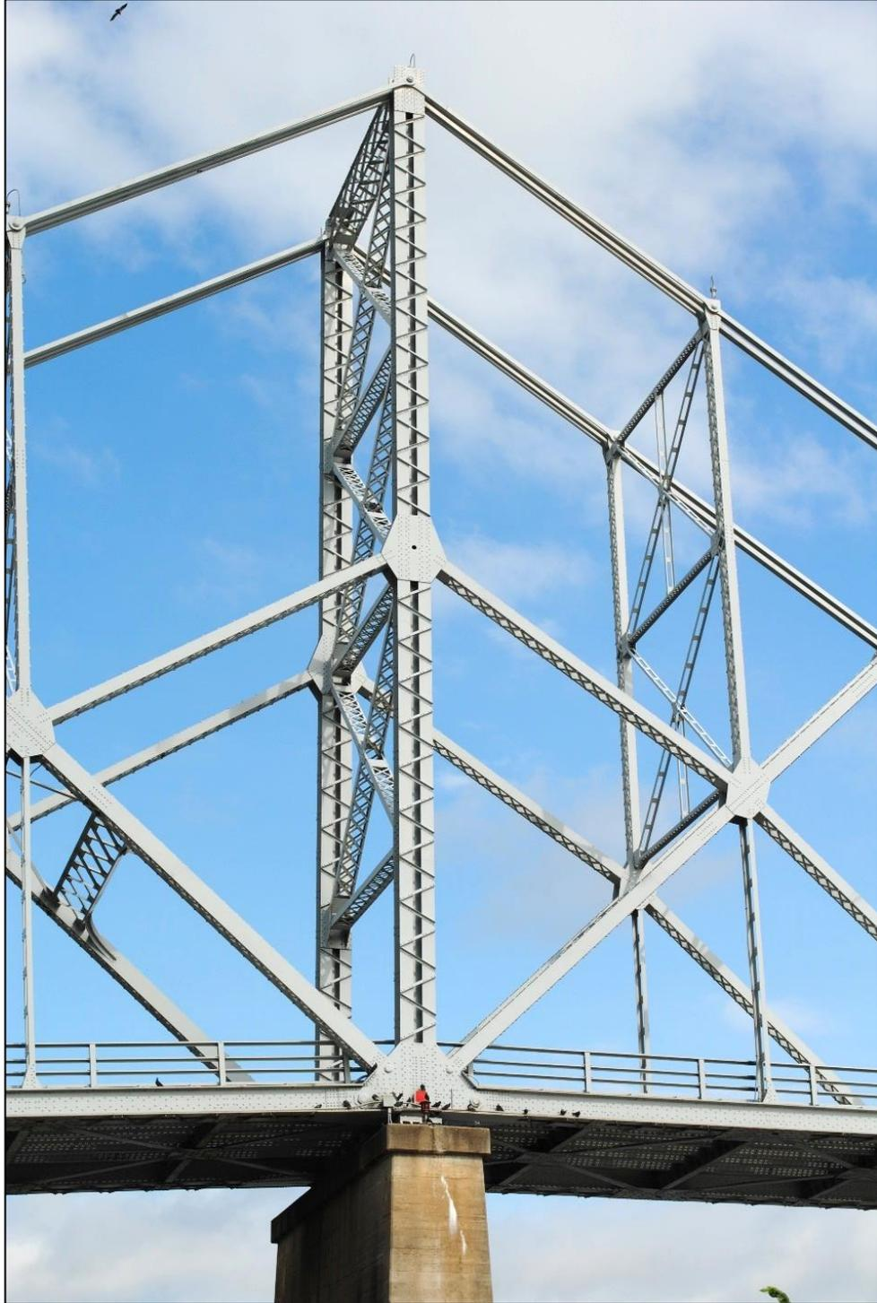
**Figure 12. Detail view of center vertical and other joints and lacing of west cantilever span peak, looking north.** Source: Tallgrass Archaeology LLC, September 18, 2022.
