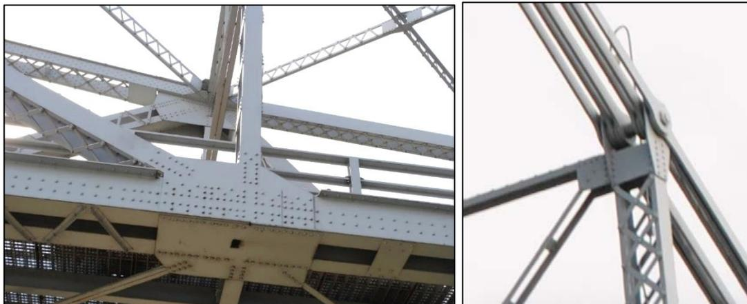
**Figure 11. Examples of superstructure connections. Left: gusset connection. Right: pin connection.** Source: Tallgrass Archaeology LLC, September 18, 2022.
