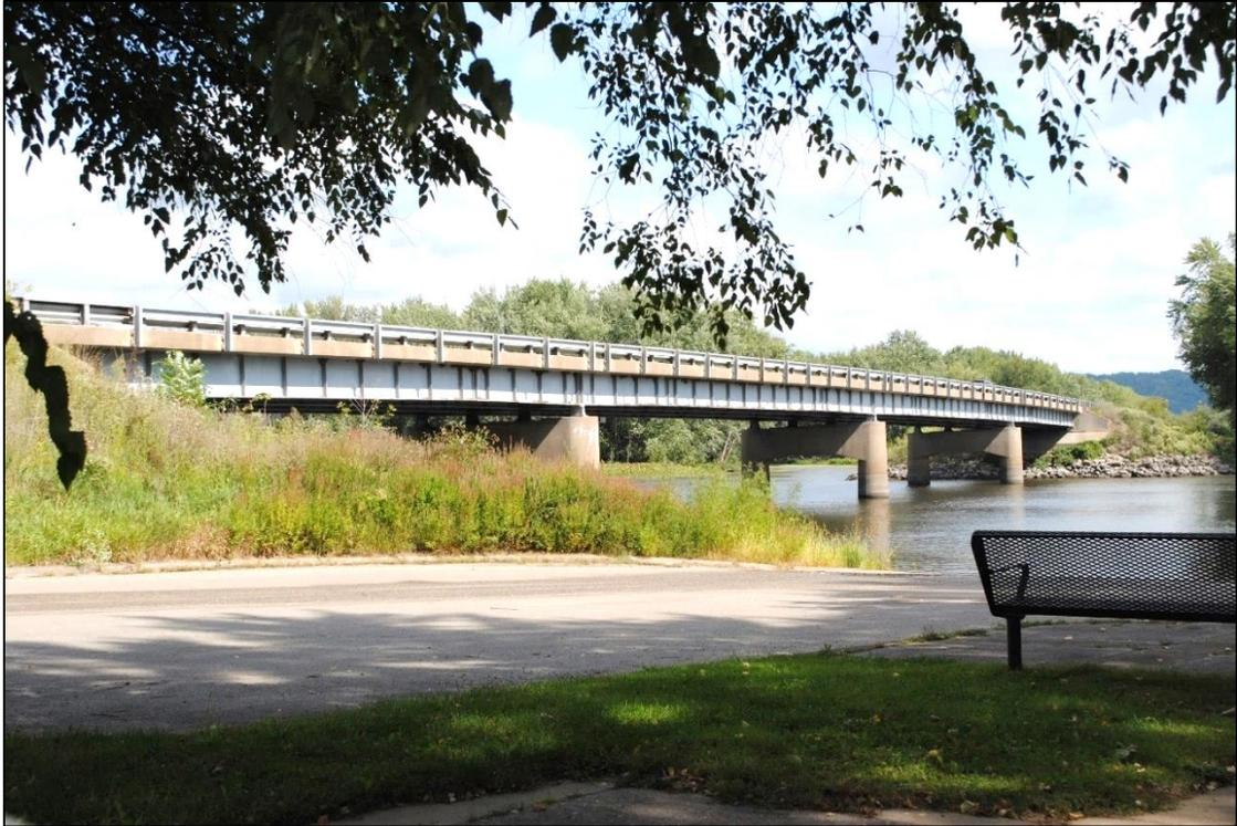
**Figure 27. West 1956 slough bridge, at Big Slough Boat Landing, looking northeast, an example of concrete and steel girder slough bridge design.**
