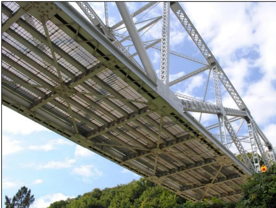
**Figure 16. View from below of steel grid deck and braces across bottom of the bridge, looking southwest under the west span. Note the visibility through the deck.**
