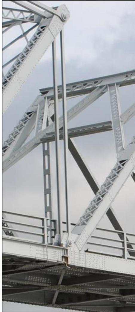
**Figure 10. Detail view of suspension-cantilever connections including pin connection, looking northeast.** Source: Tallgrass Archaeology LLC, September 18, 2022.
