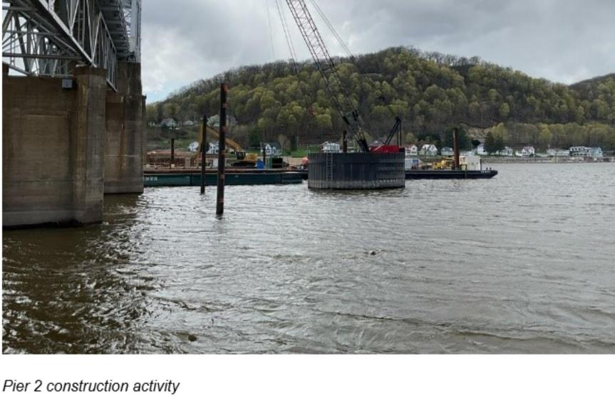
Work is also taking place in the river where pier 2 will rise from the water. This pier will also have a footing sitting on three drilled shafts. The contractor is working with a large crane on a barge getting everything ready to start drilling deep into the riverbed for these shafts.
