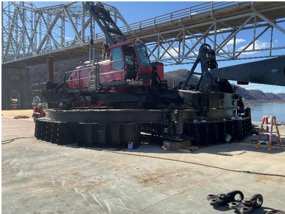
A new piece of equipment is arriving in pieces on the job site and getting put together to go to work. It's called a ringer crane because of the ring it sits on. Instead of moving back and forth on a set of tracks like most cranes, this one can rotate 360 degrees. It is being assembled on a barge and will be used in the river for construction of piers 1 and 2 as well as the new bridge.
