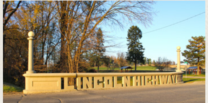
Historic Lincoln Highway Bridge in Tama County Image © 2010 Michael Kelly, all rights reserved
