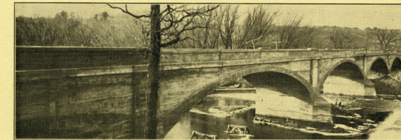
HIGH WATER WILL NOT WASH THIS AWAY Eureka Mill Bridge—On Lincoln Highway in Greene county. This bridge took the place of the structure wrecked by high water. It was built from Highway Commission plans and is of the type being built all over the state under the new road law.
