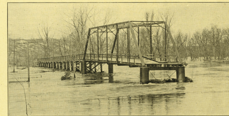
IOWA IS NOT BUILDING BRIDGES LIKE THIS NOW Eureka Mill Bridge, Greene county, on Lincoln Highway. Compare this with the concrete structure shown on another page and which replaced it.
