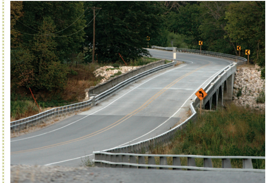
↑ The Eureka Bridge seen today from the west.
