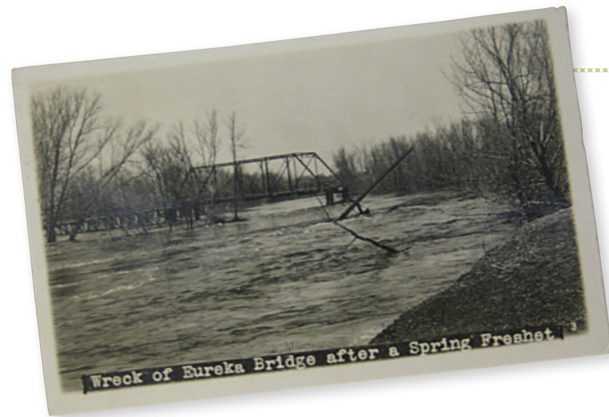
⚡ Flooding in 1912 on the North Raccoon River brought down the east span of the Eureka Bridge and precipitated planning for a new bridge design. By the end of the year, the present bridge was in place. (Iowa Department of Transportation)
