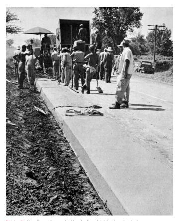
Plate 2. Slip-Form Paver in Use in Road Widening Project ISHC 1956:7
