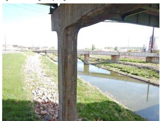
Figure 3-1. Cracking and Spalling of Pier
