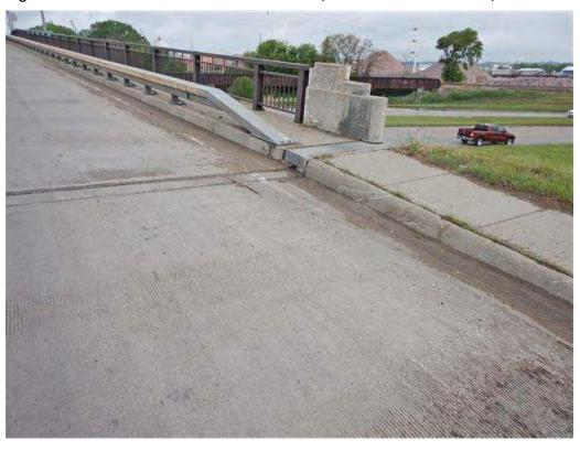
Figure 3-2. Substandard Pedestrian Sidewalk (northeast end of viaduct)
