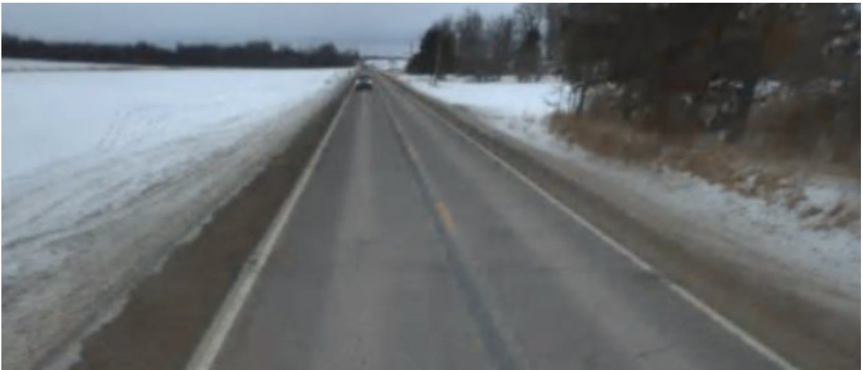
End of SB #2 Looking North
