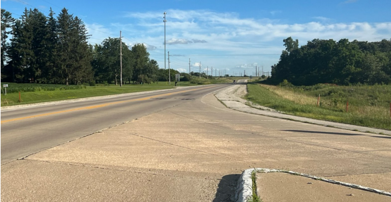
Start of SB #5 Looking South
