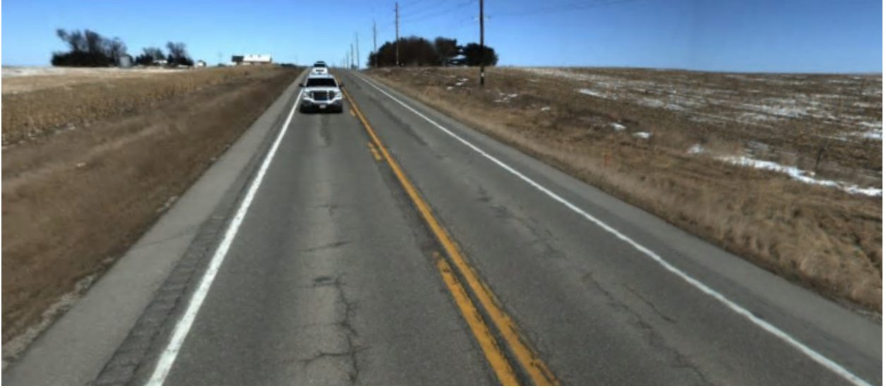
Start of NB #1 Looking North
