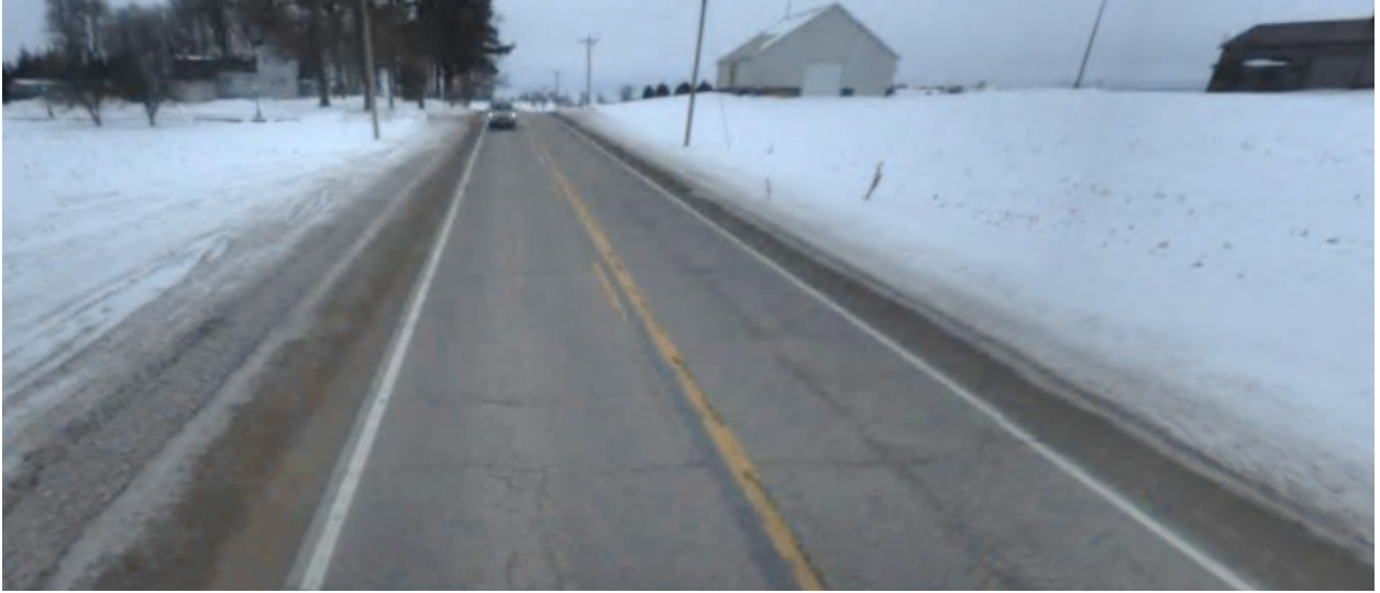
Start of NB #2 Looking North
