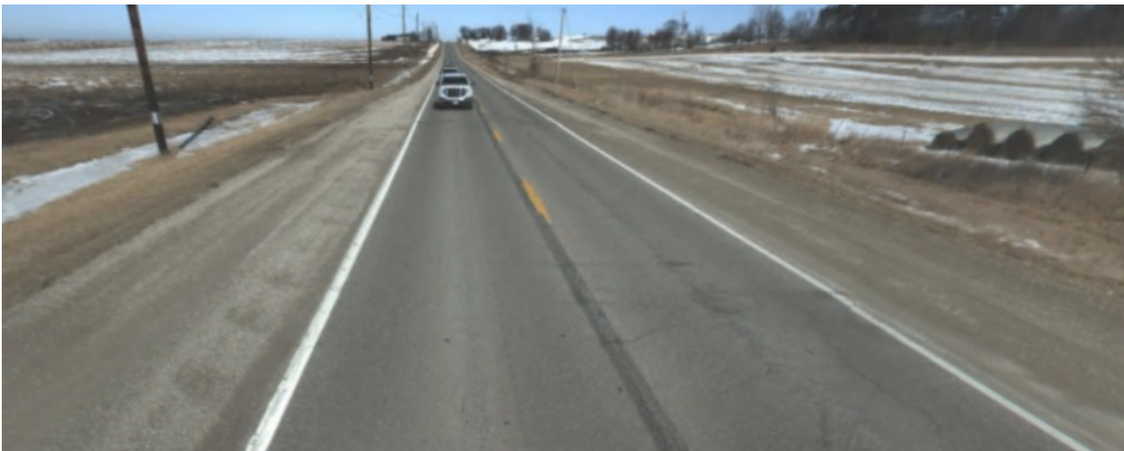
End of SB #1 Looking North
