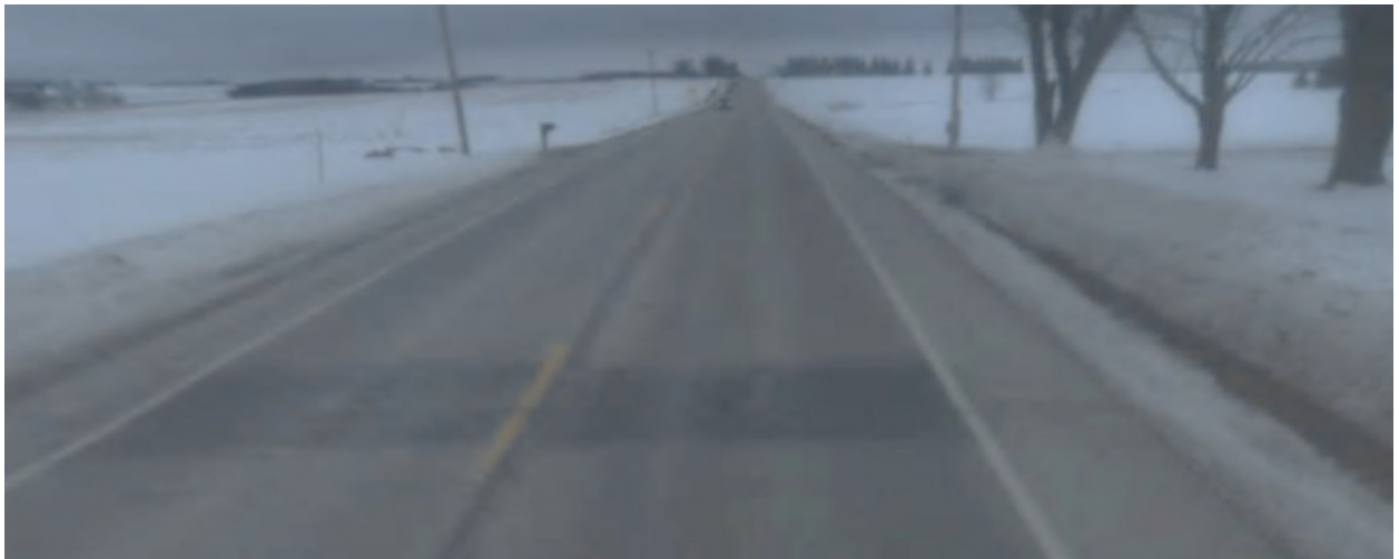
End of NB #4 Looking South
