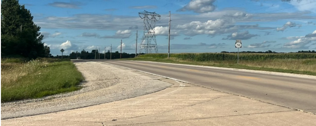
End of SB #5 Looking North
