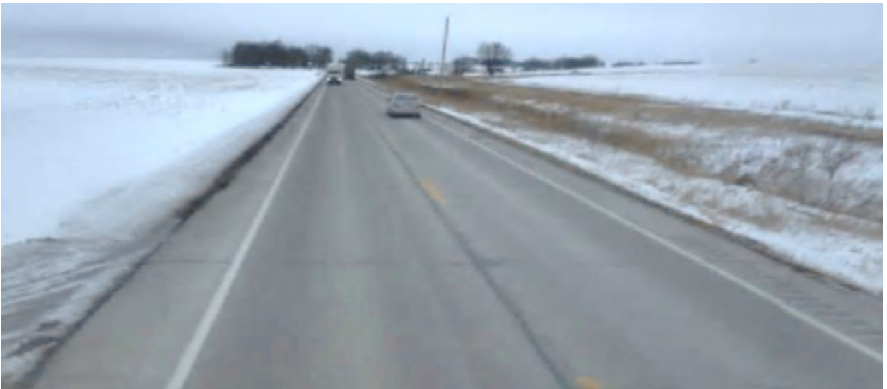
End of SB #4 Looking North
