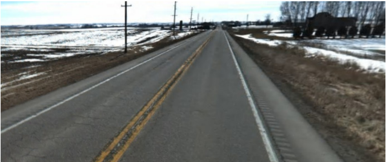
End of NB #1 Looking South
