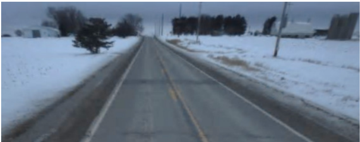
End of SB #3 Looking North
