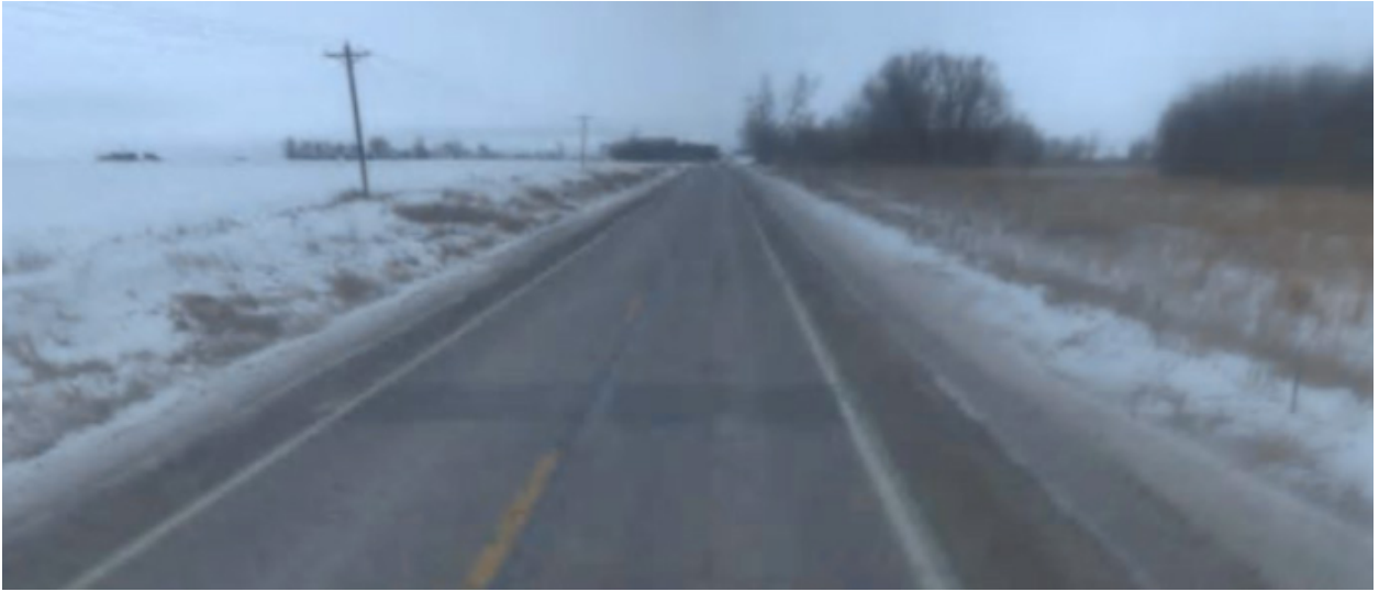
Start of SB #2 Looking South
