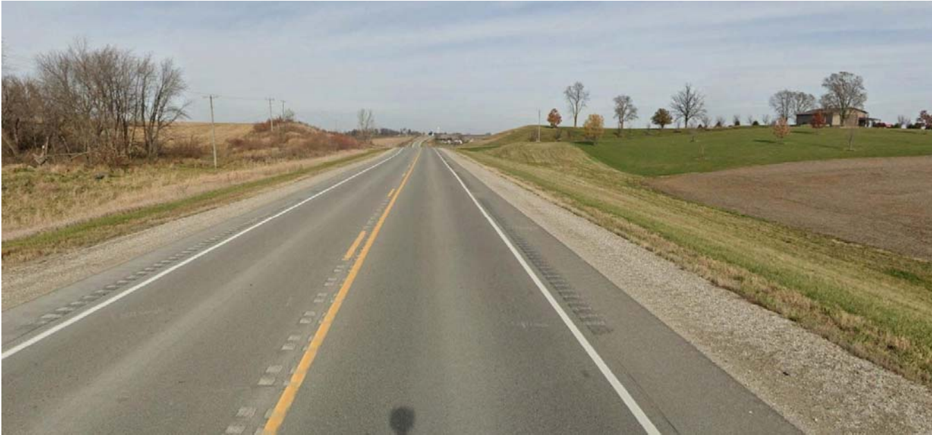
End of Existing CL #1 SB #1 Looking North
