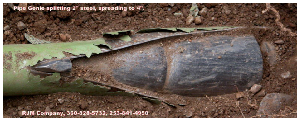
Figure 2.25. Pipe splitting (RJM Company)
