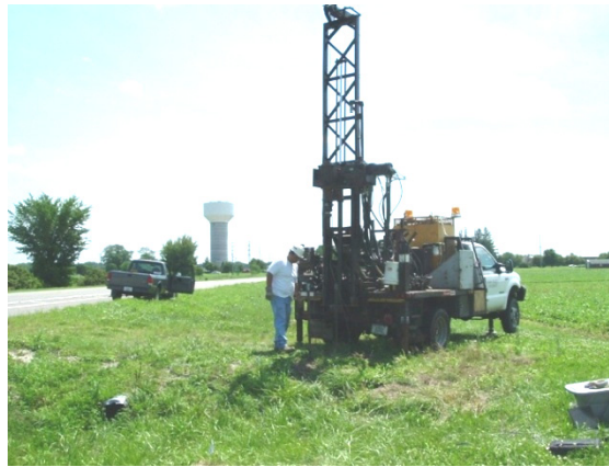
Figure 4.126. Push-in pressure cells being installed
