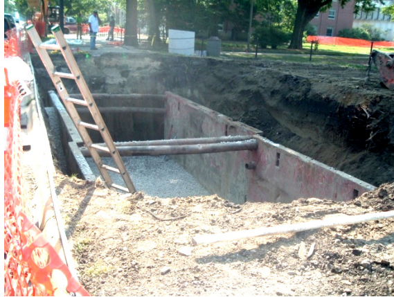
Figure D.13. Launching pit with shoring and a gravel base
