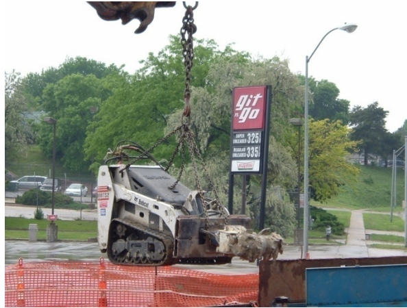
Figure 4.16. Mini road header used to excavate soil as pipe was jacked in
