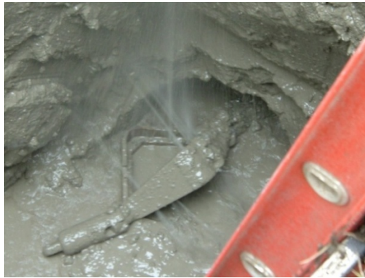
Figure 4.41. Reamer shown jetting drilling fluid in point D exit pit just before pullback
