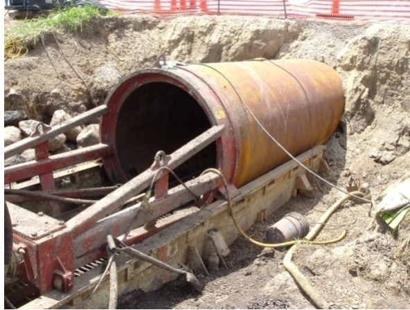
Figure 4.24. Pipe being jacked into the soil behind the TBM
