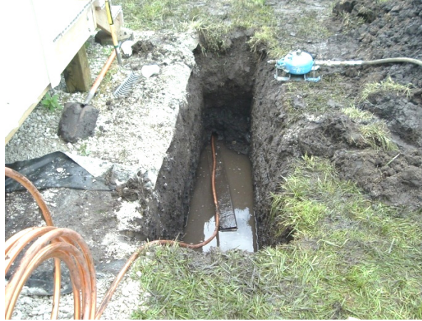
Figure 4.113. Entry pit at point A as 0.75-inch copper pipe was pulled into 2.5-inch-diameter hole
