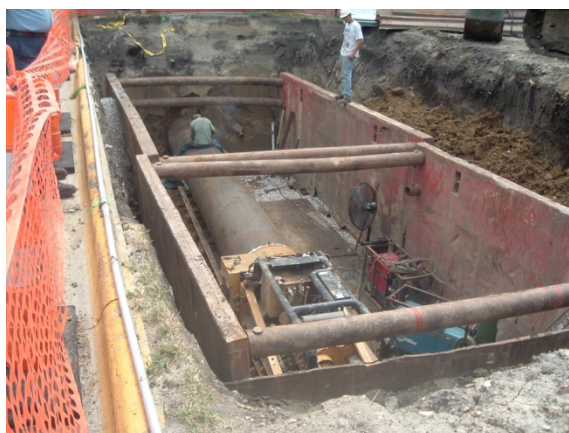
Figure D.15. First casing being bored from the launching pit
