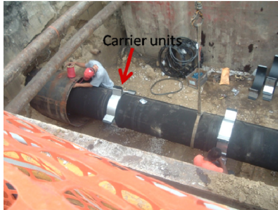
Figure D.16. The first ductile iron water pipe with casing spacers attached is placed by backhoe into the steel casing
