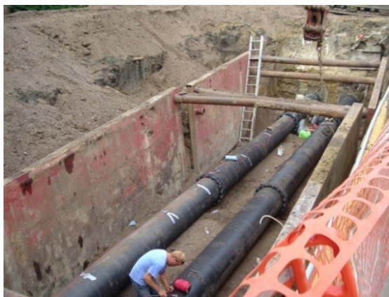
Figure D.18. The final connection of pipe sections in the launching pit
