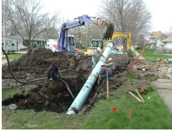
Figure D.47. Sixteen inch pipe being lowered into the exit pit at point B, before it is pulled into place by the drill rig
