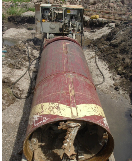
Figure 2.6. Rotating cutter head TBM
