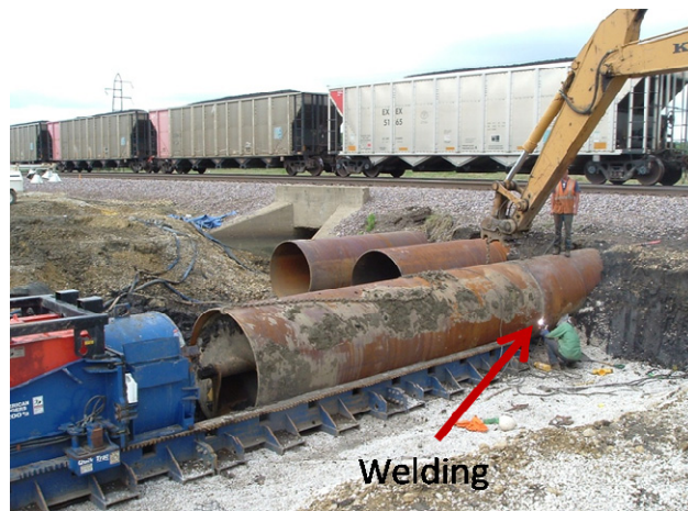
Figure D.28. A new 20 foot long pipe section being welded to the pipeline
