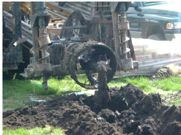
Figure D.46. Twenty-four inch wagon wheel reamer
