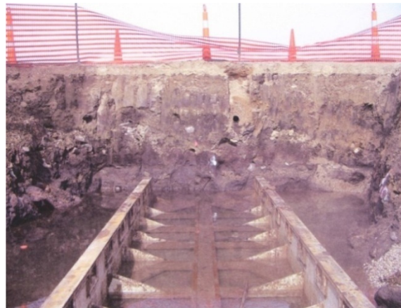
Figure 4.20. Partially flooded launching pit at point A, with track installed prior to tunneling
