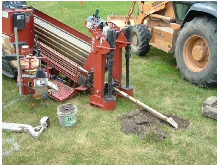
Figure 2.11. Pilot bore being started by pushing drill bit into soil
