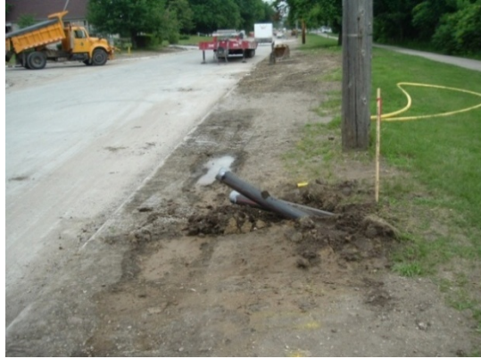
Figure 4.43. Capped 4-inch HDPE pipes after installation at point E next to Beach Avenue
