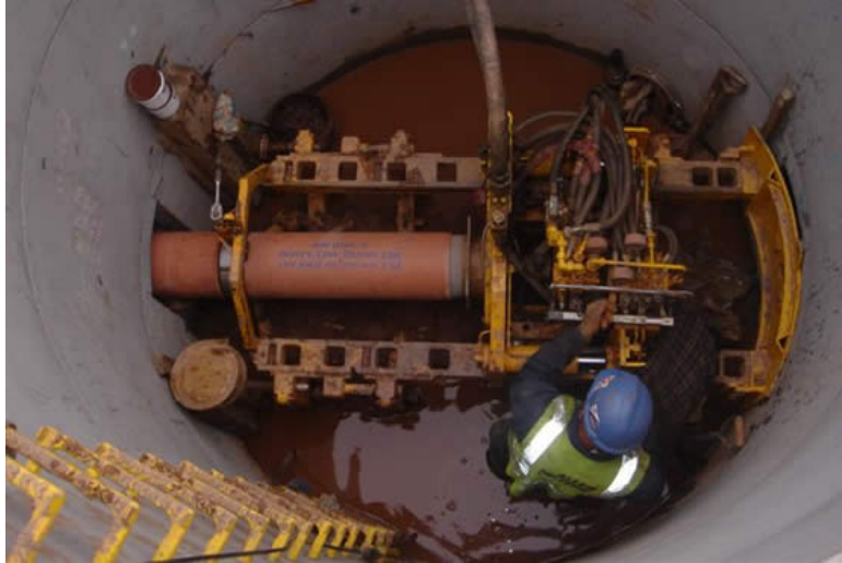
Figure 2.5. Vitrified clay pipe being installed using guided auger boring (from Allen Watson, Ltd.)
