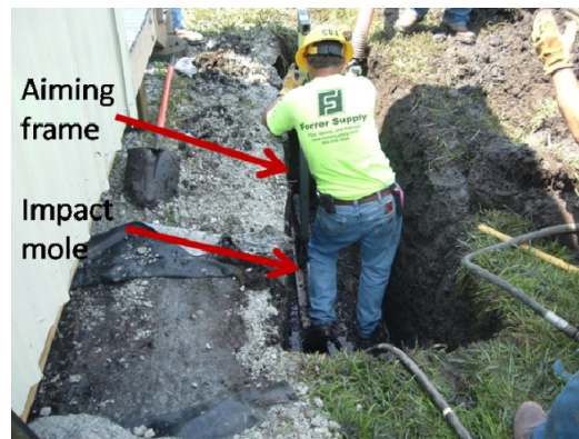
Figure 4.110. Launching the mole and adjusting line and grade using telescopic aiming frame
