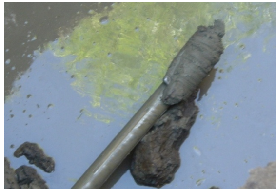
Figure 4.53. Clay-caked drill bit shown after emerging into the exit pit at point D
