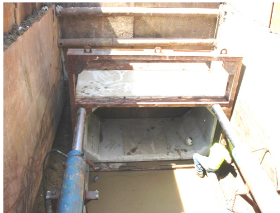
Figure 4.15. Jacking begins on the first box pipe section
