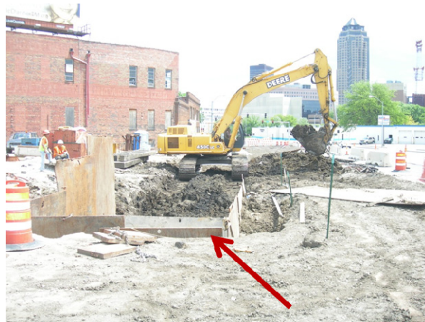
Figure 4.12. Launching pit with trench box and steel plates
