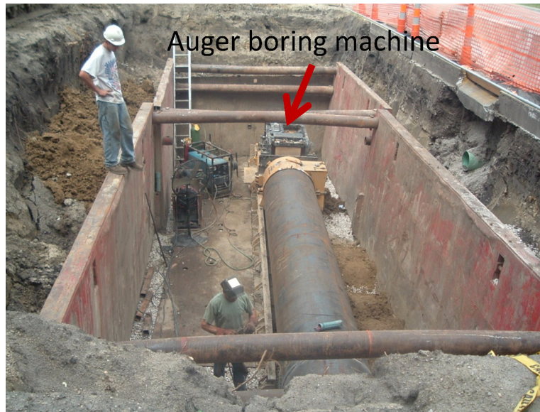
Figure 2.2. Launching pit with auger boring machine installing pipe
