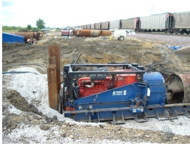
Figure D.27. Auger boring machine on its track against the sheet pile thrust block
