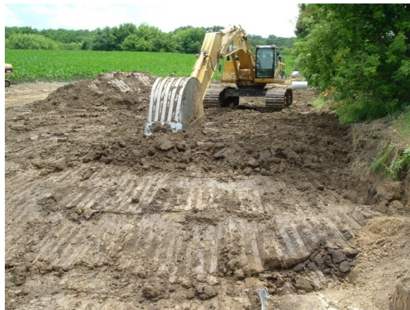
Figure D.5. Launching pit at point A being filled in as the installation is completed
