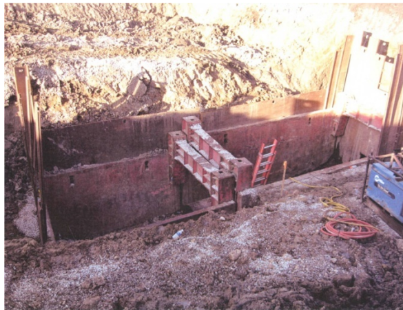
Figure 4.29. Launching pit with shoring and gravel base
