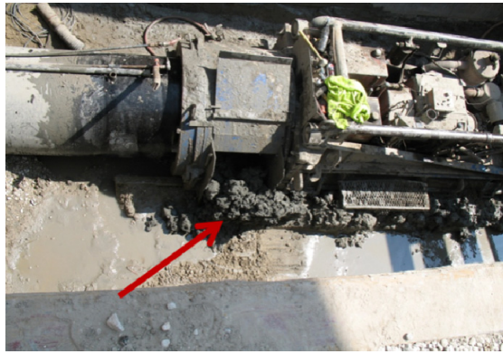
Figure 4.7. Clayey weathered shale deposited out of auger boring machine
