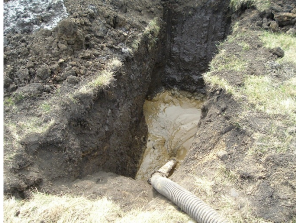
Figure D.38. Drilling fluid being vacuumed from the bottom of the exit pit at B
