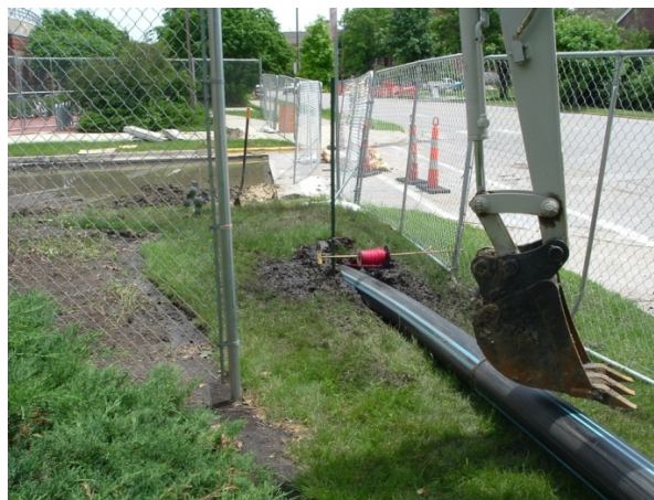
Figure 4.102. HDPE pipe (8-inch diameter) pulled into borehole at point A
