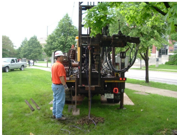
Figure 4.103. Installing push-in pressure cell
