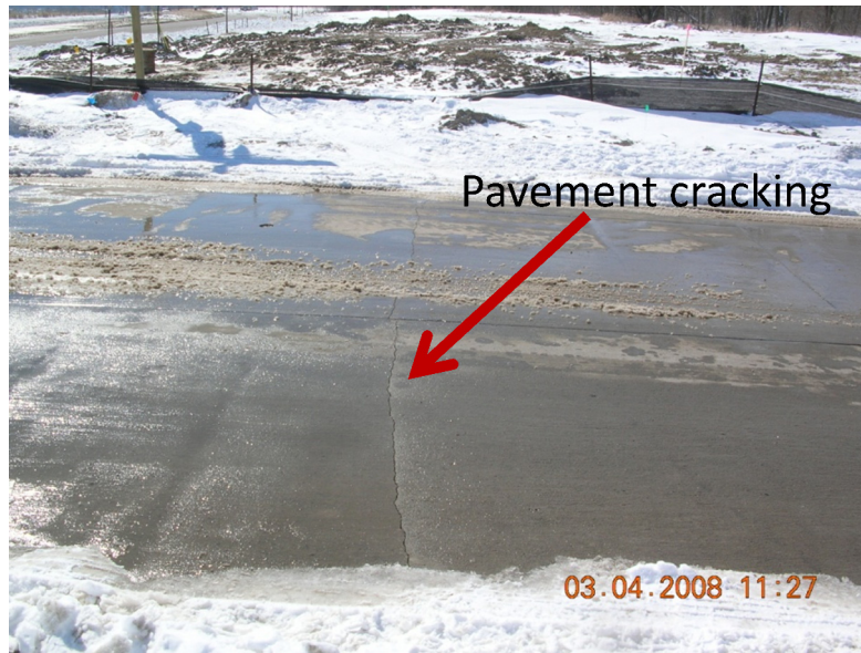
Figure 3.15. Pavement cracking caused by HDD installation
