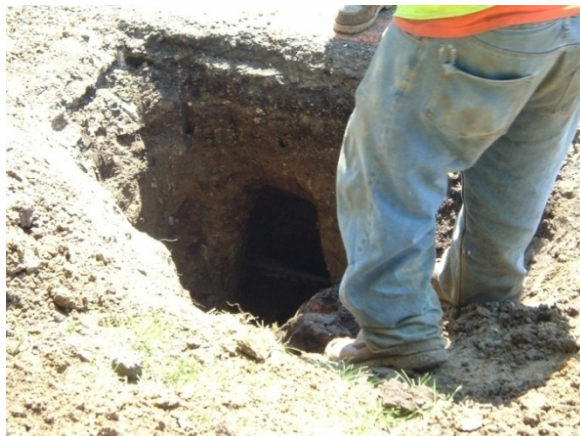
Figure D.2. Potholing by edge of pavement
