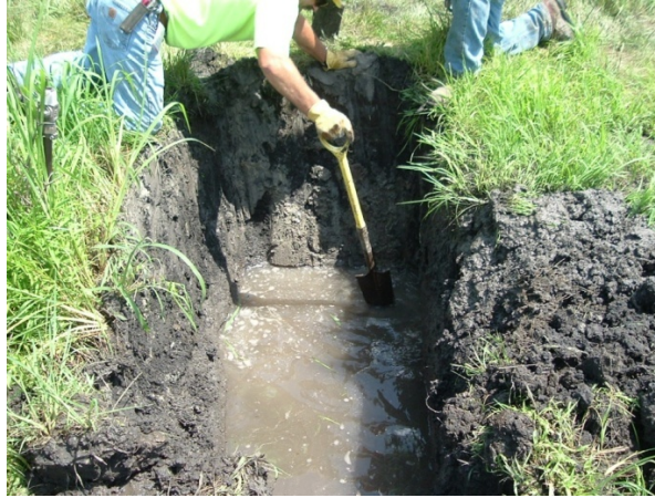
Figure 4.111. Locating mole after it emerged at point C into exit pit, which was flooded
