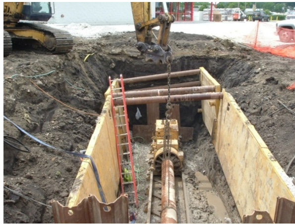
Figure D.10. A backhoe lowers a new 20 foot section of steel pipe into the launching pit
