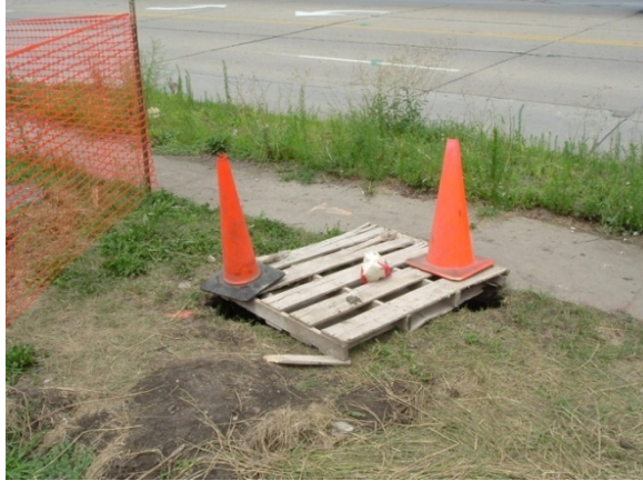
Figure D.9. A potholing pit covered and marked
