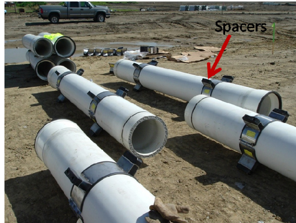
Figure 4.32. PVC carrier pipe with visible spacers
