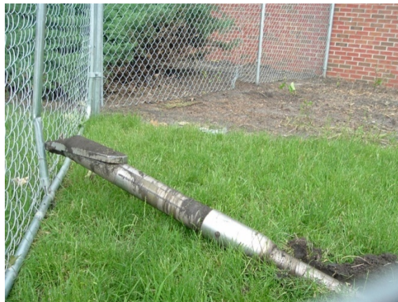
Figure 4.100. Drill bit (5-inch diameter) emerging at point A
