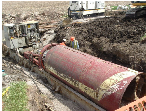
Figure 4.21. TBM before starting the bore
