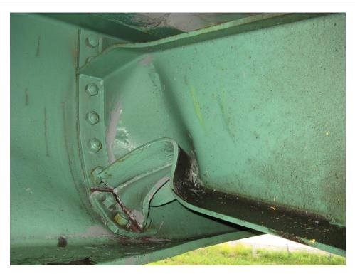
Figure 2.9.3.1-3. Damaged Diaphragm Member
