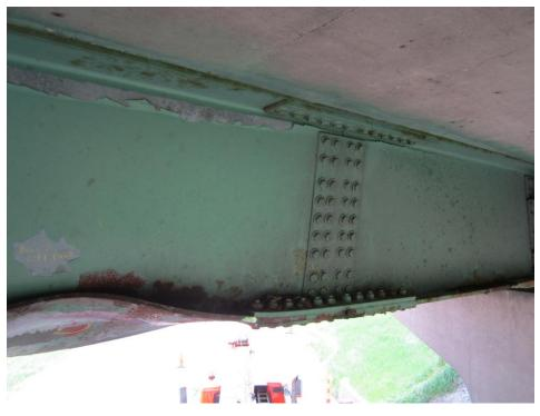
Figure 2.9.3.1-2. Moderately Bent Bottom Flange with Some Web Distortion
