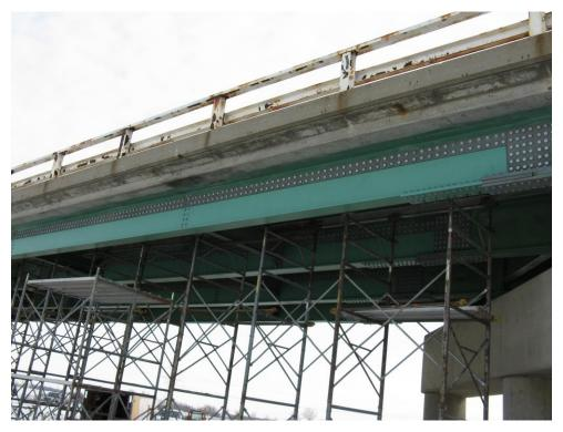
Figure 3.2. Partial Steel Beam Removal and Replacement
