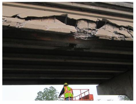
Figure 2.9.3.2-6. Severe Prestressed Beam Damage with Excessive Concrete Section Loss
