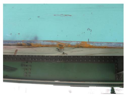
Figure 2.9.3.1-1. Steel Gouge and Paint Scrape
