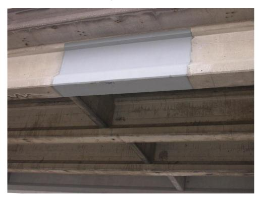
Figure 4.2. Fiber Reinforced Polymer Wrapped Repair
