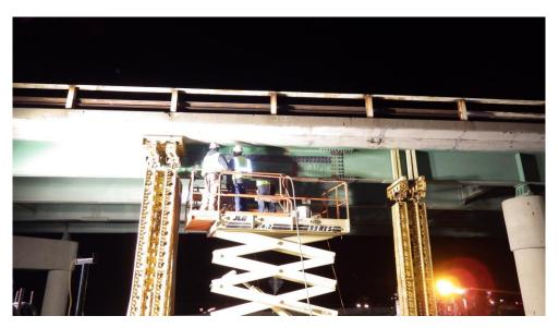
Figure 3.4-1. Shoring Towers on Each Side of Damage
