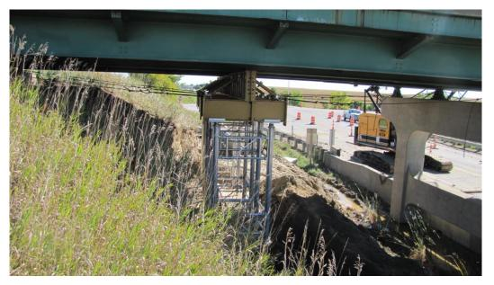
Figure 3.4-2. Shoring Tower Providing End Span Support
