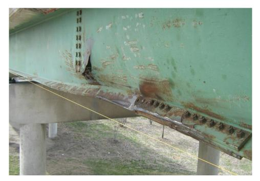
Figure 2.9.3.1-4. Out of Plane Bending with Web Tear
