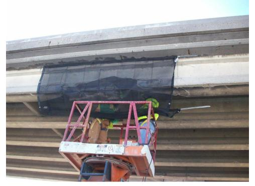
Figure 2.9.3.2-1. Installation of Drape to Catch Loose Debris
