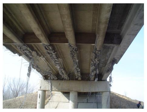
Figure 2.9.3.2-7. Multiple Prestressed Beams with Severe Damage
