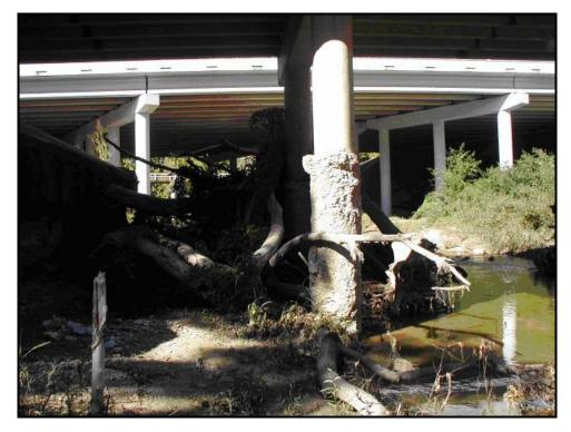
Figure 5.1.4. Bridge Pier Scour Damage
