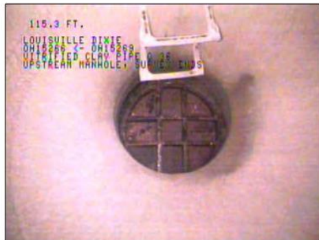
Photo: OH15269_OH15266124956_05112009_A.JPG, VCR No.: FLOOD WALL#2, 01:47:25 115.3FT, Upstream Manhole, Survey Ends
