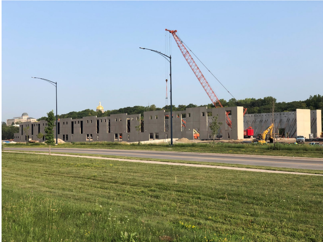
View from Martin Luther King Jr. Parkway looking NW
