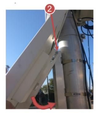
2) Install PMG to Pole Bracket via preinstalled bolt on PMG. Then Rotate into position
