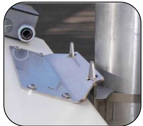
Installed Top Bracket
